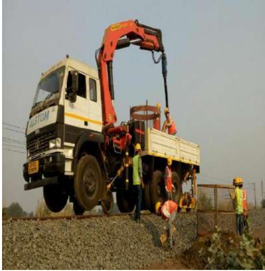
Foundation auguring by rail based mobile augur
