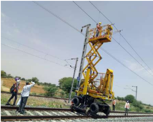
Mechanized inspection of works using rail borne vehicles such as Vertical Cradle Platform (VCP) and tower wagon etc.
