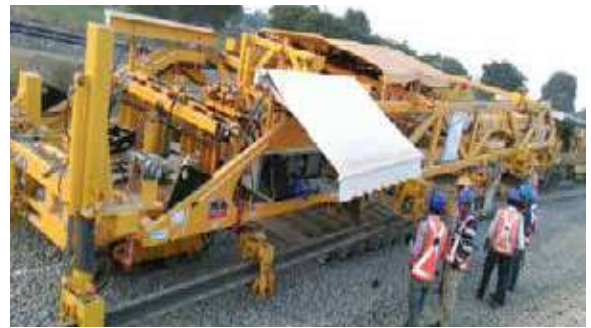
Track linking work in Progress
