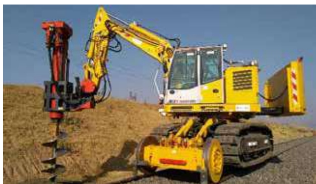
OHE Foundation Auguring by Colmar
