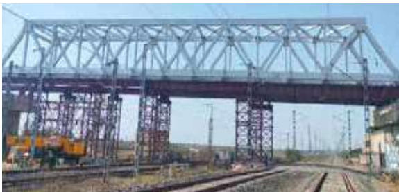
Open Web Girder of 71.1 m on LC 161 was launched on 07.06.2023 in Palanpur-Makarpura Section of WDFC.
