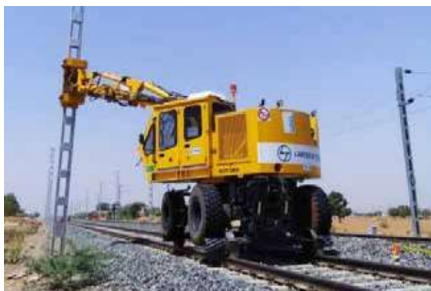
Mast Erection by Mast Grabber
