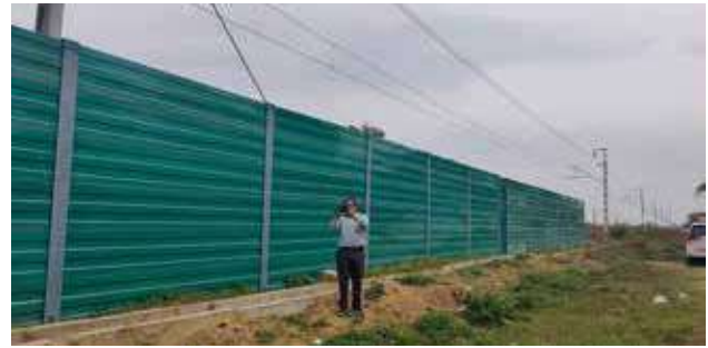
Installed Noise Barrier at Lot 303
