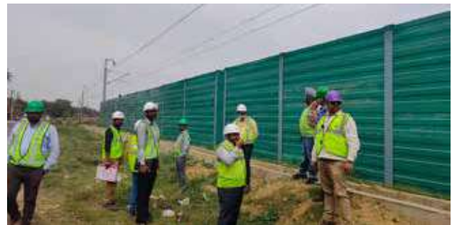
Noise Barrier Inspection by World Bank at Lot 303
