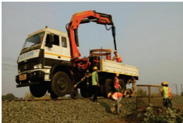
Foundation auguring by rail based mobile augur
