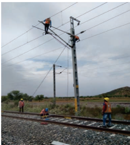
Contactless SED checking using infrared system for accuracy in measurement & minimal human involvement
