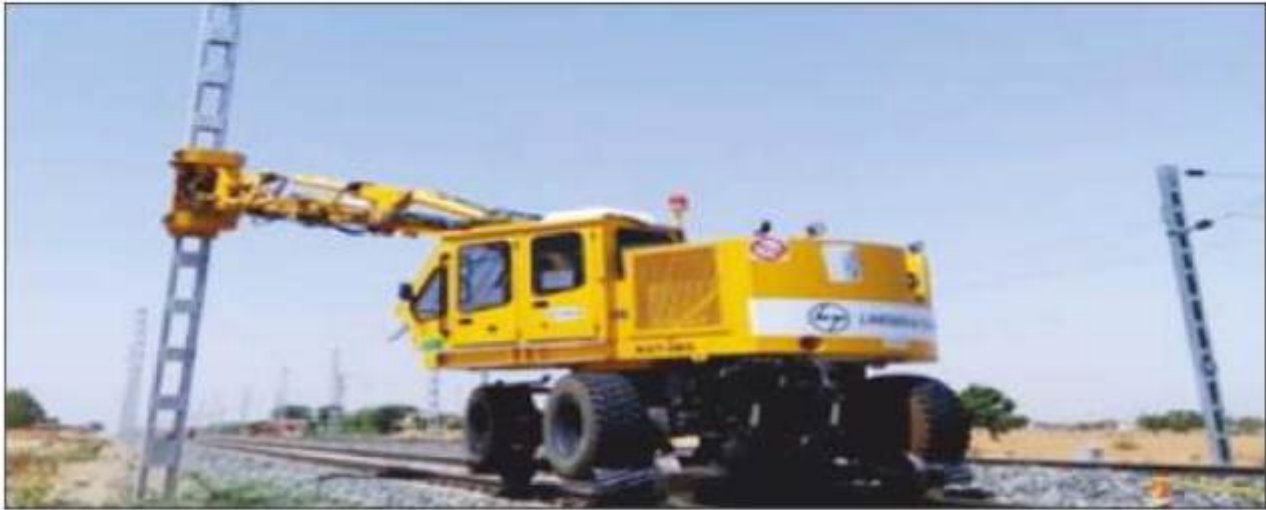
(Mast Erection by Mast Grabber)
