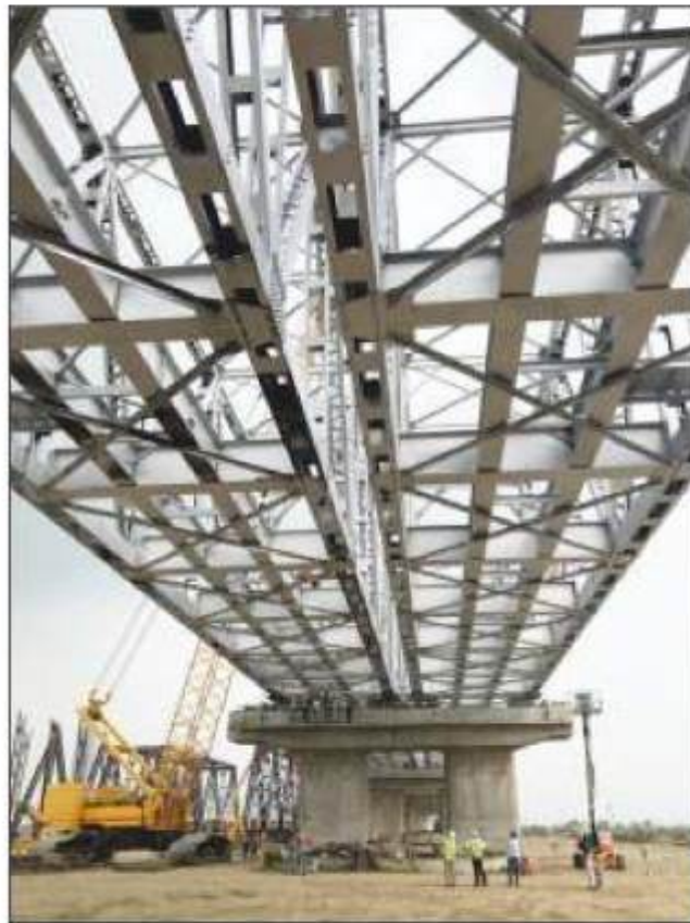
Launching of girders on bridge over Yamuna in Rewari-Dadri section
