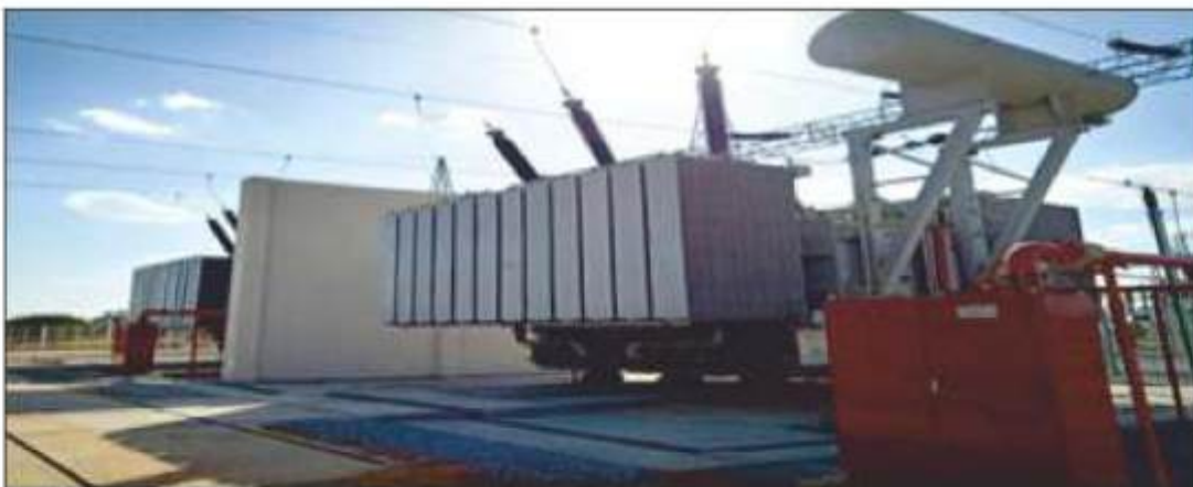
(Scott Transformer & NIFPS System at Ringus TSS, Rajasthan)
