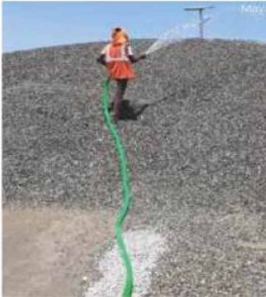
Reuse of wastewater in dust suppression
