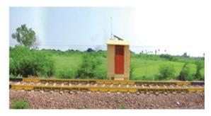
Hot Axle Hot Wheel Detector (HAHW): It detects axle box and wheel tread which are running abnormally hot and measures the temperatures as well. It detects the same up to a speed of 100 Kmph of rolling stock. It automatically transmits data, alarms and reports to the end users.
