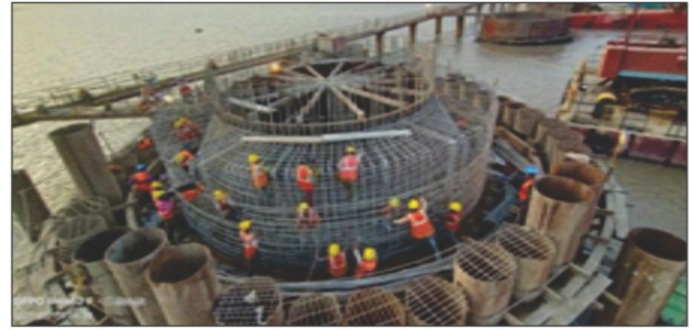
Fig.3 (b) Well Curb ell Curb Reinforcement
