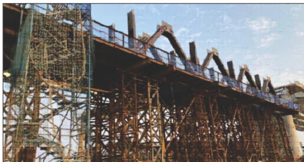
Fig.8: P28-P27 Assembly of Girder on Trestles
