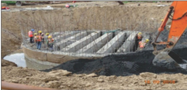
Fig.4(a) Cutting edge –Water well
