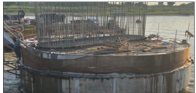
Fig.5(b) Well Cap Casting
