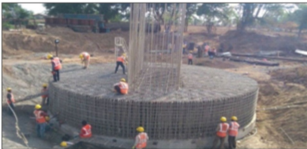
Fig.5(a) P2- Well Cap Reinforcement
