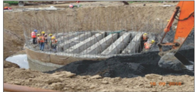
4 (b) Well Curb ell Curb Reinforcement
