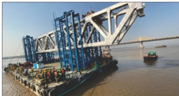
Fig.9(b) Towing of Loaded Barge with Tog Boats of 450HP
