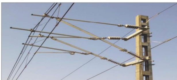
Fig. 14 : Modular Cantilever Assembly
