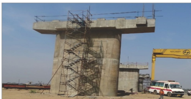
Fig.6(a) Pier P10-P11 with Pier cap
