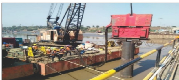
Fig.2(a) Liner Driving Vibro Hammer
