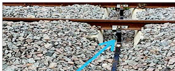
Fig. 4: Rail clamp for bonding of Rails used in DFC project
