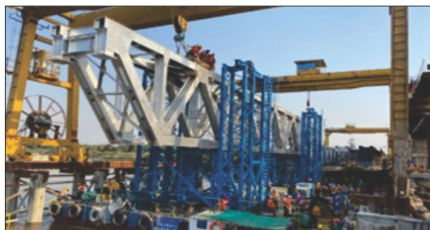
Fig 9(a): Loading of Assembled Girder on Launching Barge
