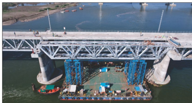
Fig.9(d) last Girder (P13-P14Up) launched on 17.10.2022
