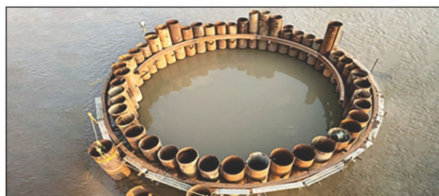
Fig.2(b) Cofferdam liner piles completed
