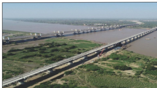
Narmada Bridge (29x48.15m) Under Slung Steel Girder with RCC Deck Slab Fig 1: Bird's eye view of Narmada Bridge No 57
