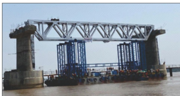
Fig.9(c) First Girder for Water Span launched on 03.03.2022
