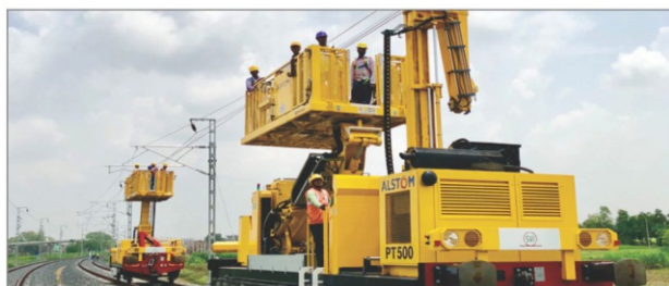
Fig. 15: Mechanized maintenance of OHE
