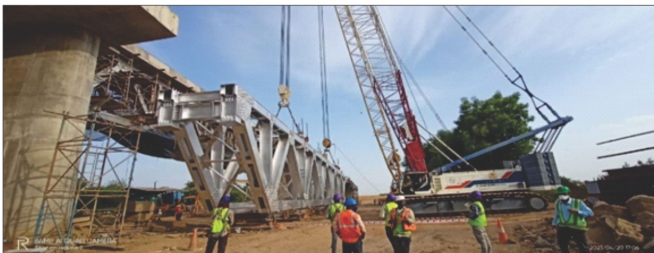
Fig.7 Launching of Under Slung Girder of 48.15m Span (130MT Wt) by tandem Lifting with two cranes (300MT & 260MT)
