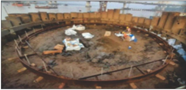
Fig.3(a) Cutting edge –Water well
