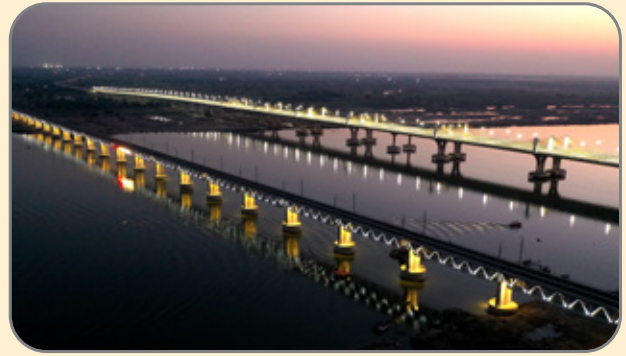
Aerial view of the Narmada River Bridge on the WDFC
