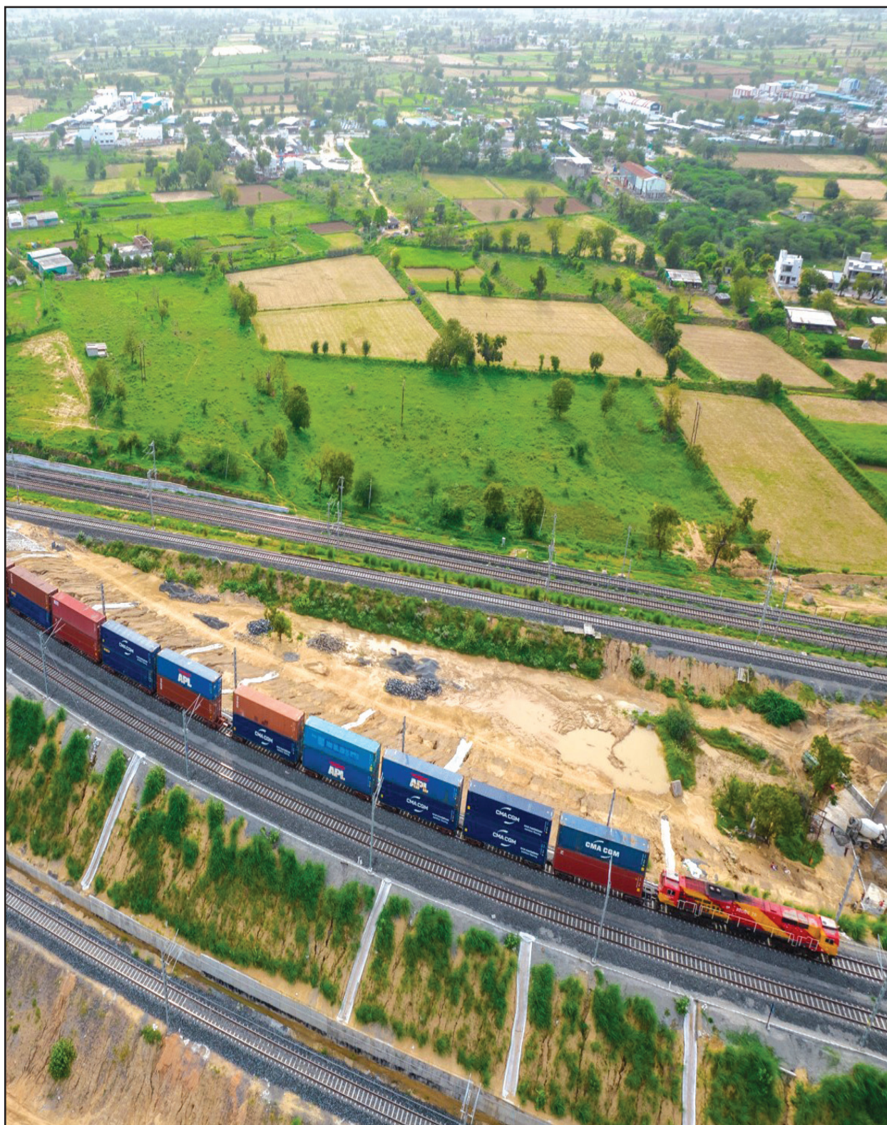
Rail Flyover (RFO-25) at Banaskantha on Palanpur Connecting Lines in New Palanpur- New Makarpura Section of WDFC
