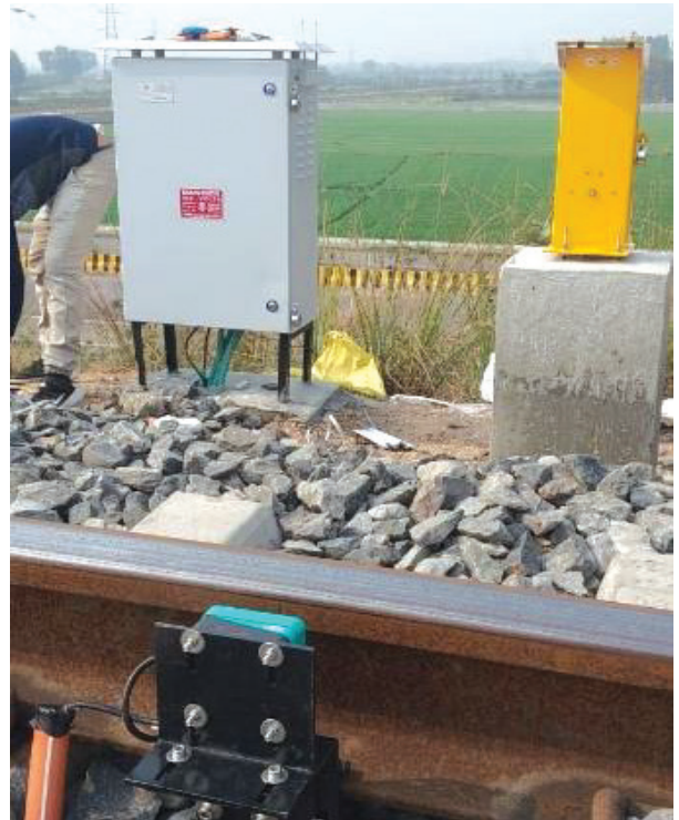
Installation of HABD on DFC Track
