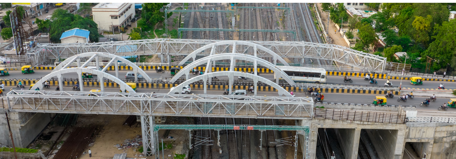
Aerial View of Twin ROB, Palanpur (WDFC)
