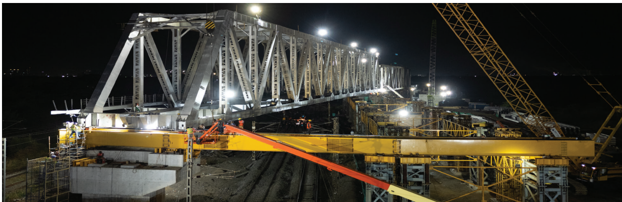
Girder Launching in Progress
