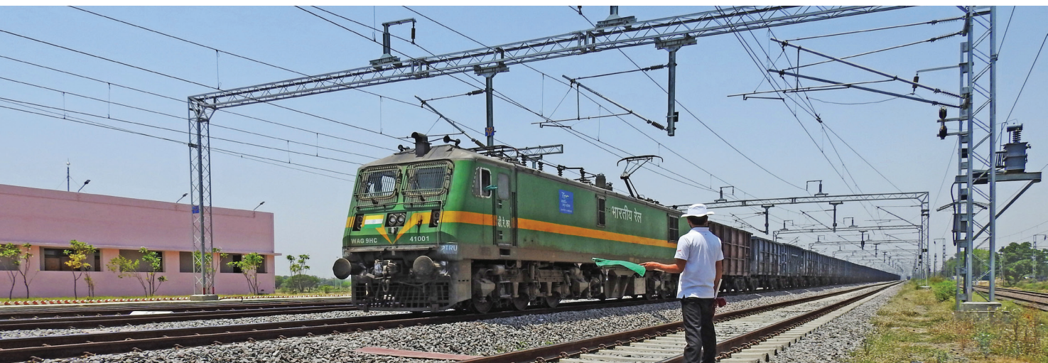
Train passing through New Manauri Station of EDFC
