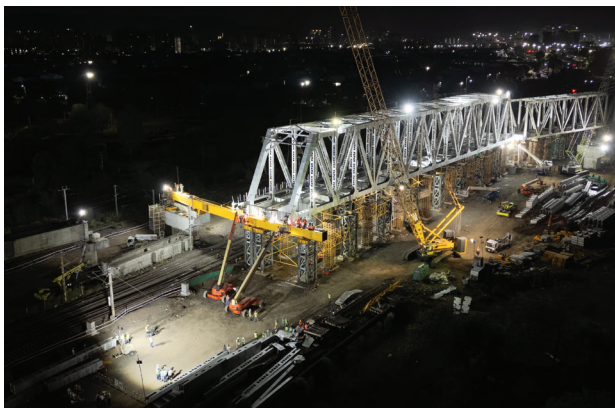
Girder Launching initiated
