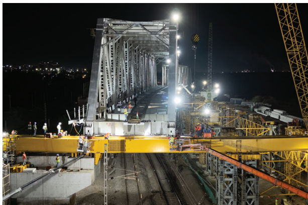
Girder Successfully Launched
