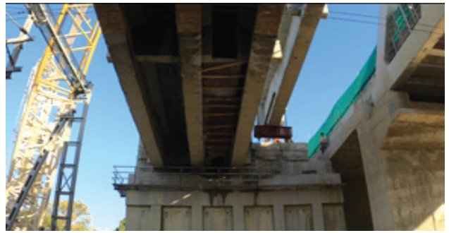
Dismantling of existing PSC Girder
