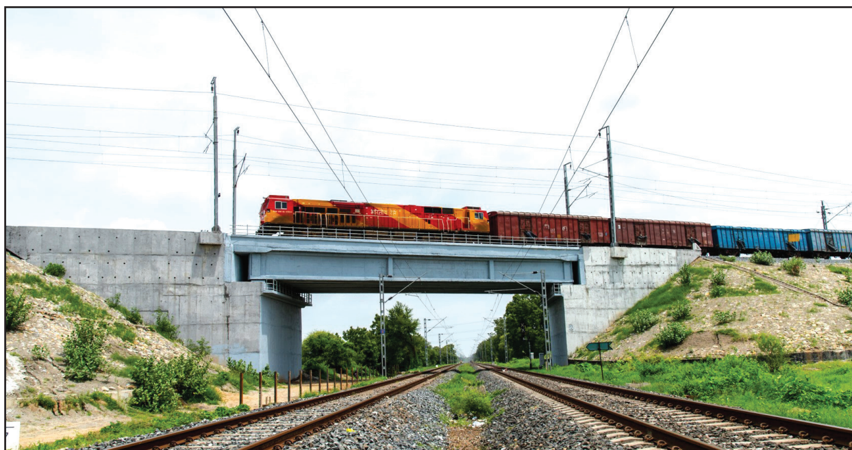
Freight train passing over Rail Flyover No. 86
