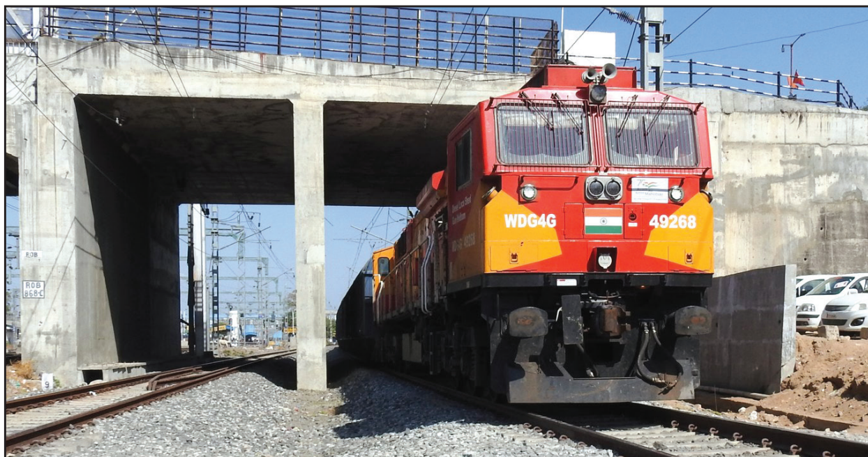
Freight train traversing the twin-box ROB at Palanpur.
