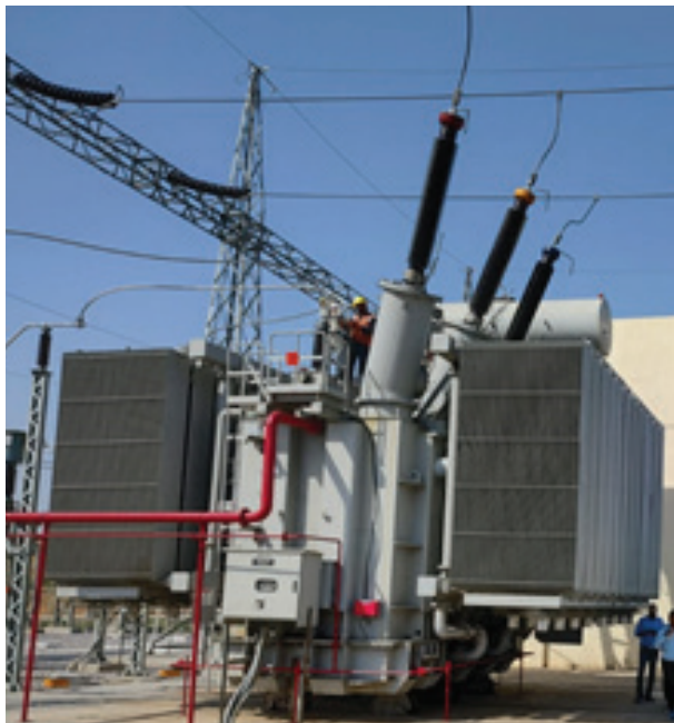
Scott Connected Transformer at one of the Sub-Station
