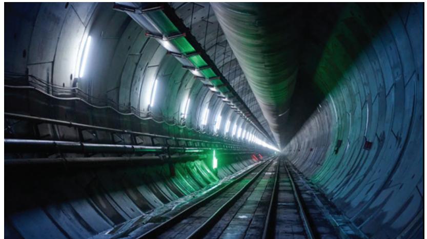
Inside view of Brenner Base Tunnel
