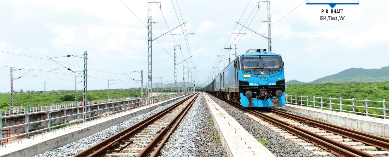
12000 HP Loco Plying through WDFC
