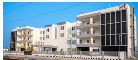
Integrated Crew Lobby and Running Room, New Palanpur
