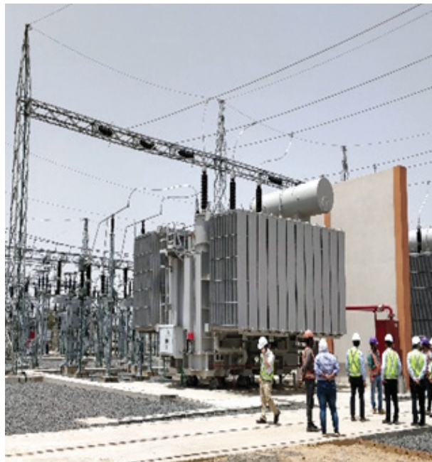
Scott Connected Transformer at one of the Sub-Station
