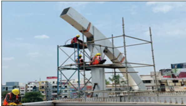
Assembling of BSG
