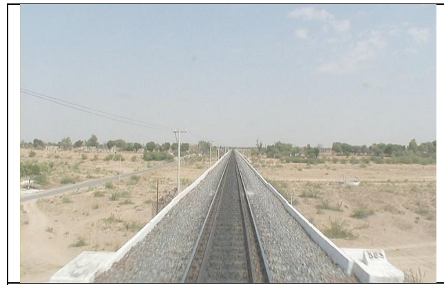
(4) River, Sojat Rd. North
