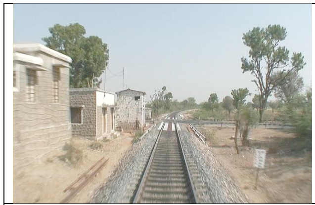
(4) NH8, Daurai South ROB (under construction)
