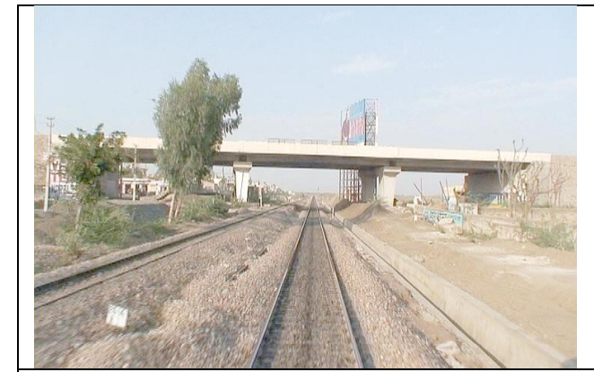
(7) NH8 Bypass, Kishangarh
