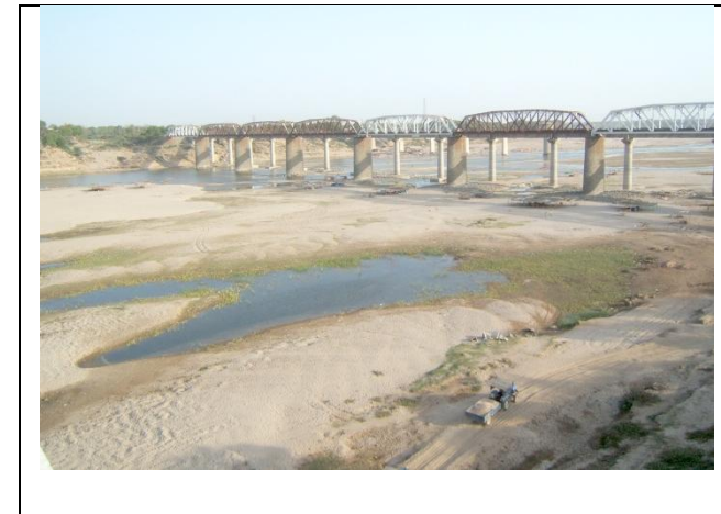
(4) Existing Railway Bridge across Mahi River (Upstream of the proposed bridge location)
