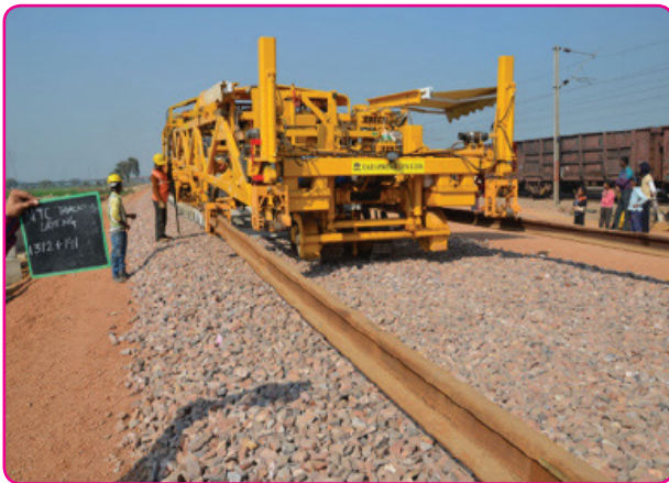
EDFC- Track laying work by NTC machine in progress
