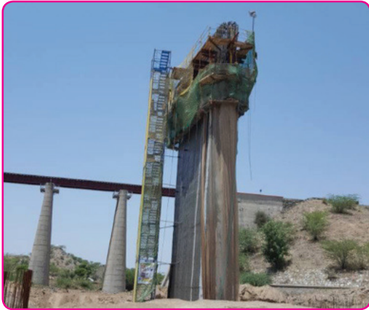
CTP-2 – Construction of 30 m high Piers of Major Bridge no. 490 by Slipform shuttering
