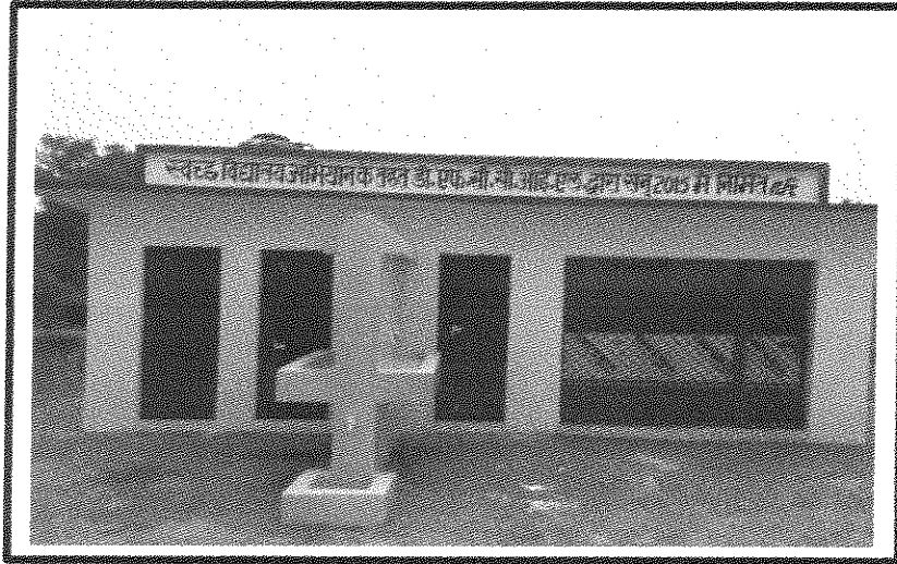
Toilet Blocks constructed under Eco-Sanitation/ Swacch Vidayalaya Campaign.
