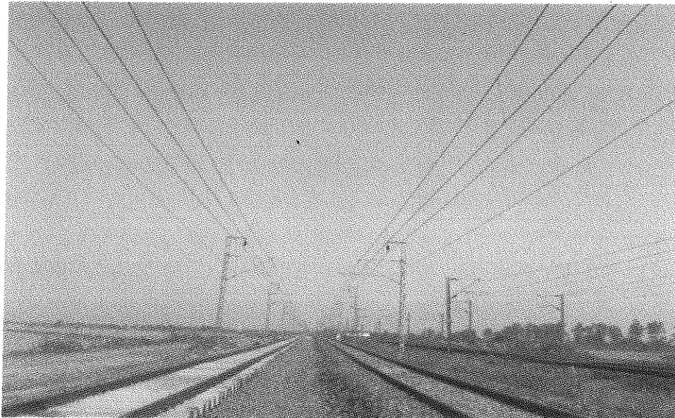
NEWLY LAID DFC TRACKS
