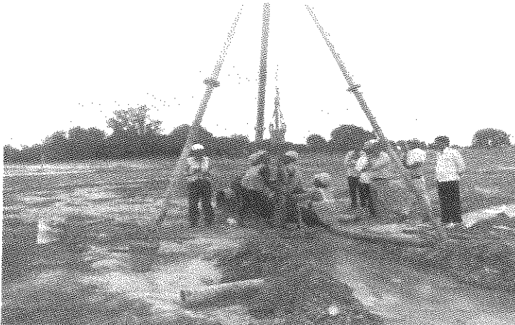
Geotechnical Investigation in Progress
