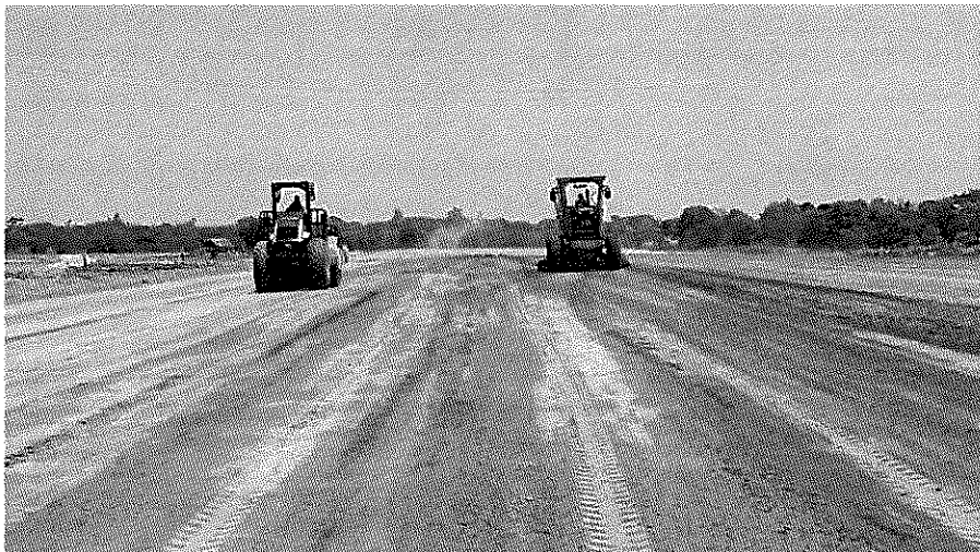
Earthwork in Mirzapur Detour
