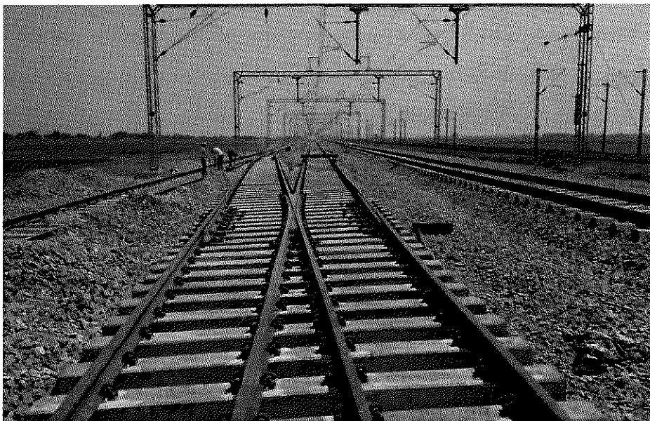
Laying of canted turnouts in Mughalsarai-Sonnagar section
