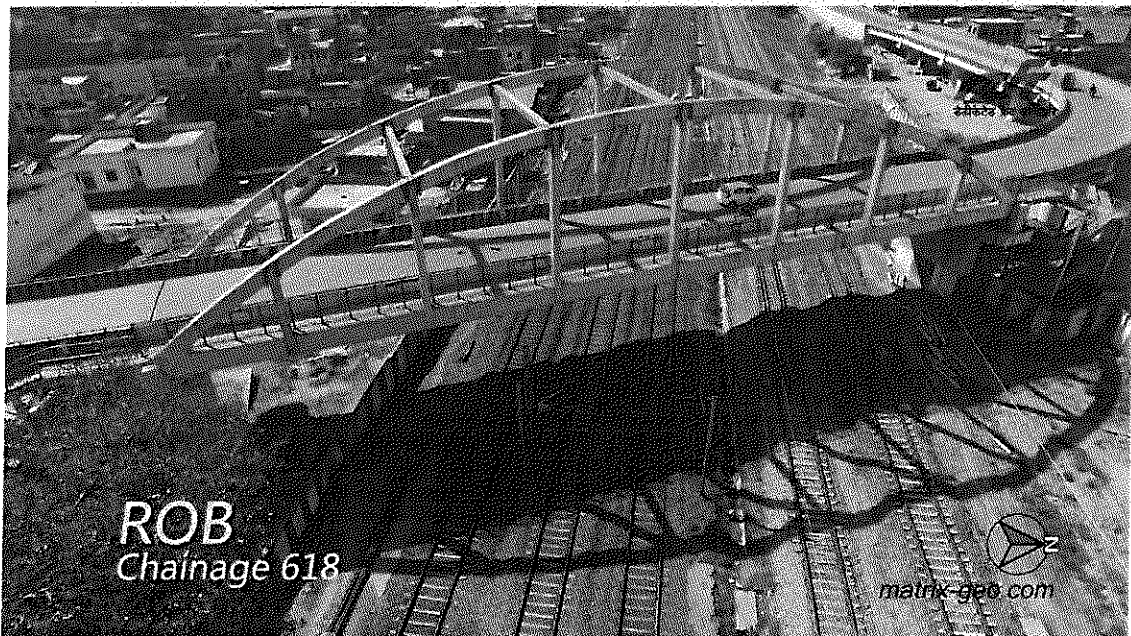
EDFC- 1 -- Work at Major Bridge in progress
