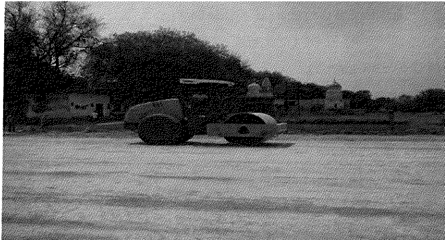
Compaction of Earthwork
