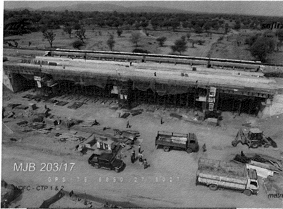
WDFC - Work at Major Bridge no. 203 in progress
