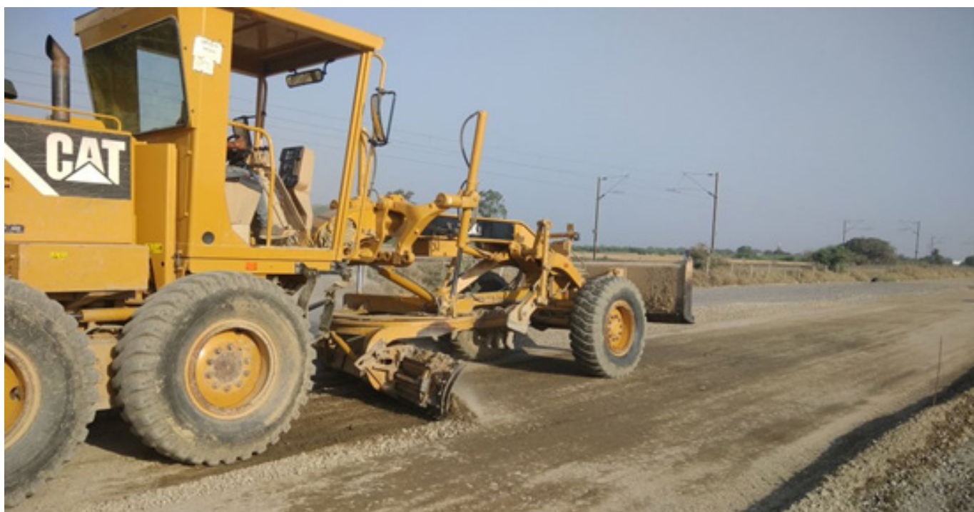
BLANKET TOP-460+900 TO 460+960 GRADING IN PROGRESS
