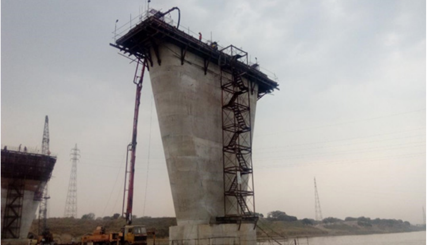
CONCRETING OF PIER CAP P13 COMPLETED
