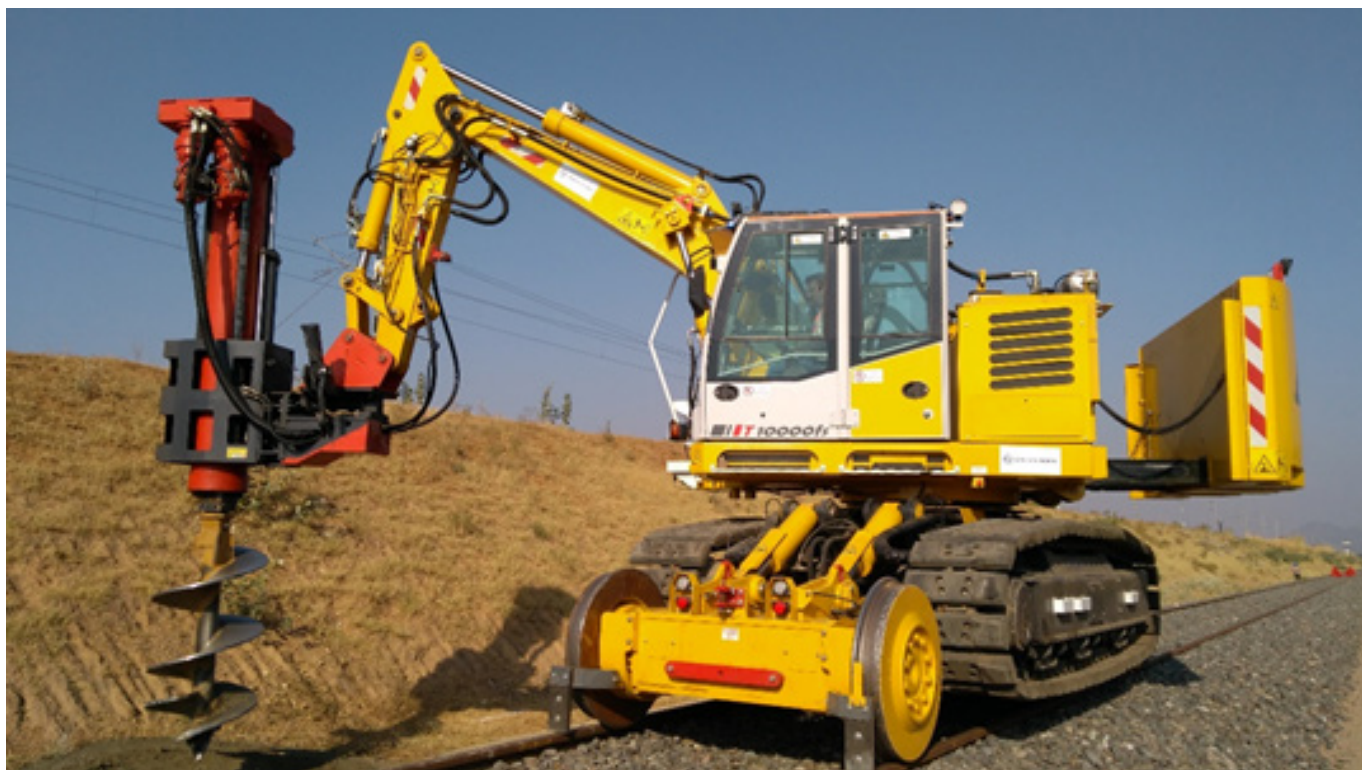
WDFC – Cylindrical Foundation Auguring in progress
