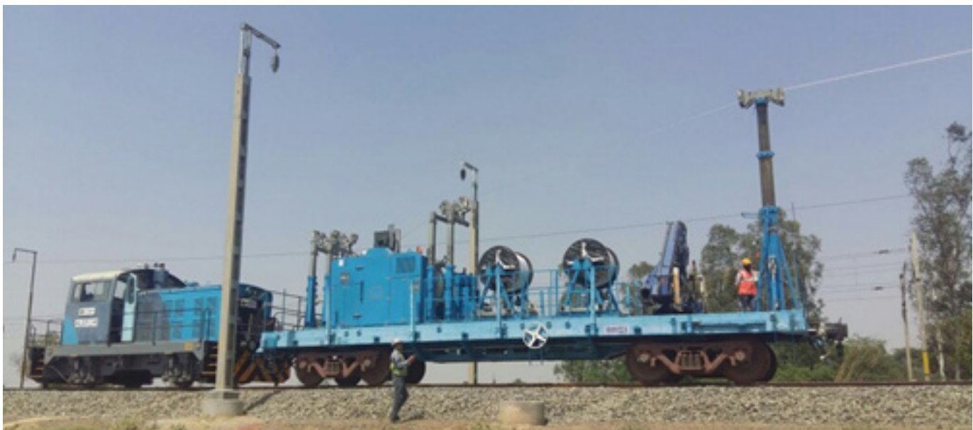
EDFC – Mechanized wiring through wiring train in progress
