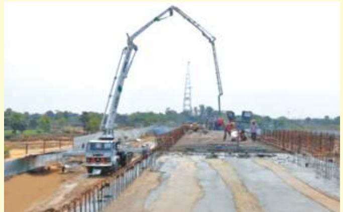
EDFC- Concreting of Girder at Sone Bridge
