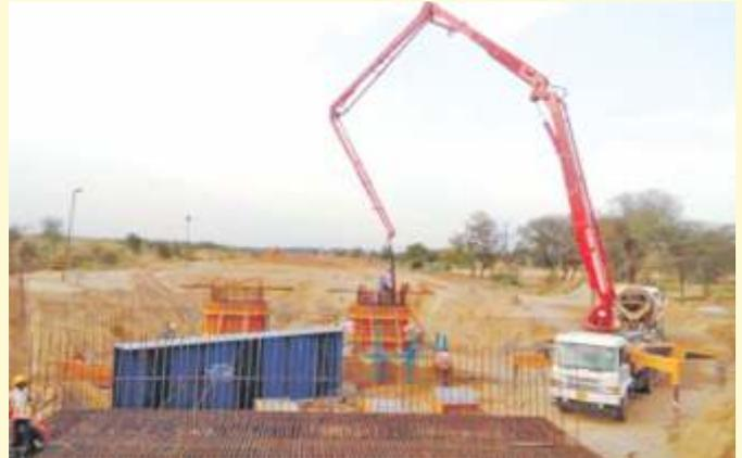
WDFC- Pier concreting Major Bridge no. 19 in progress in CTP-1
