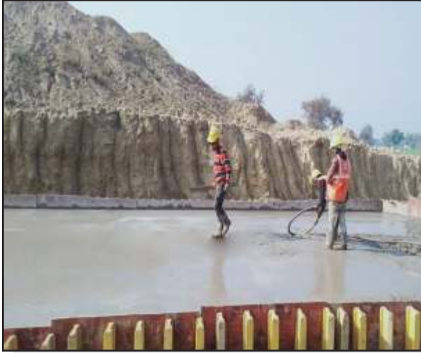
Slab casting in progress at Bridge no.144B
