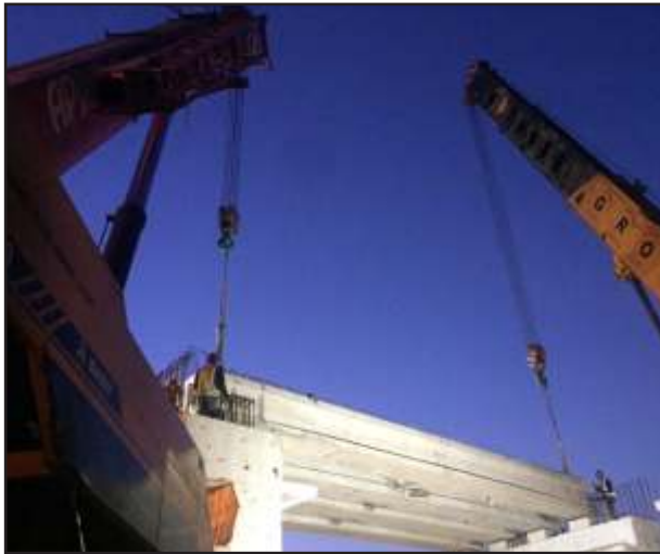
Launching of PSC Girder (Br. no. MTC19) in Khurja- Saharnpur section.
