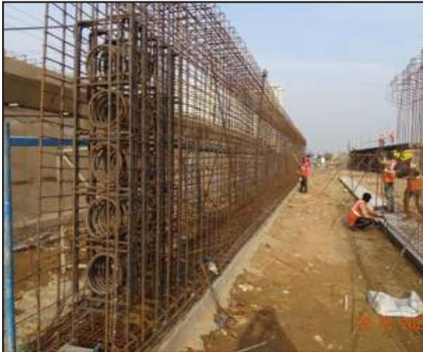
Girder Reinforcement at Dadri Casting Yard
