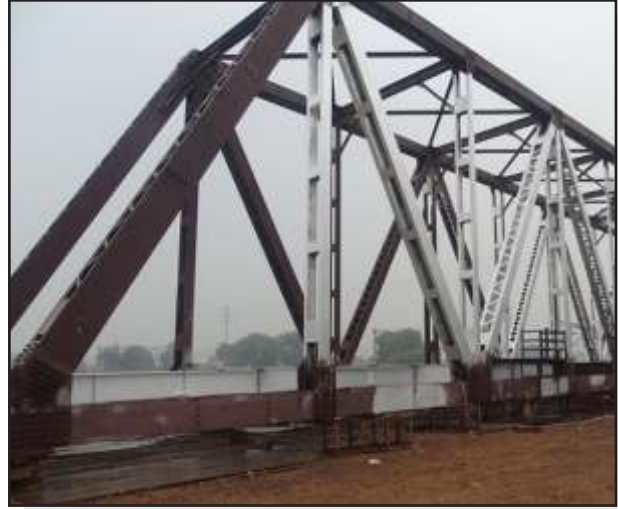
RFO Girder Final Coat Painting
