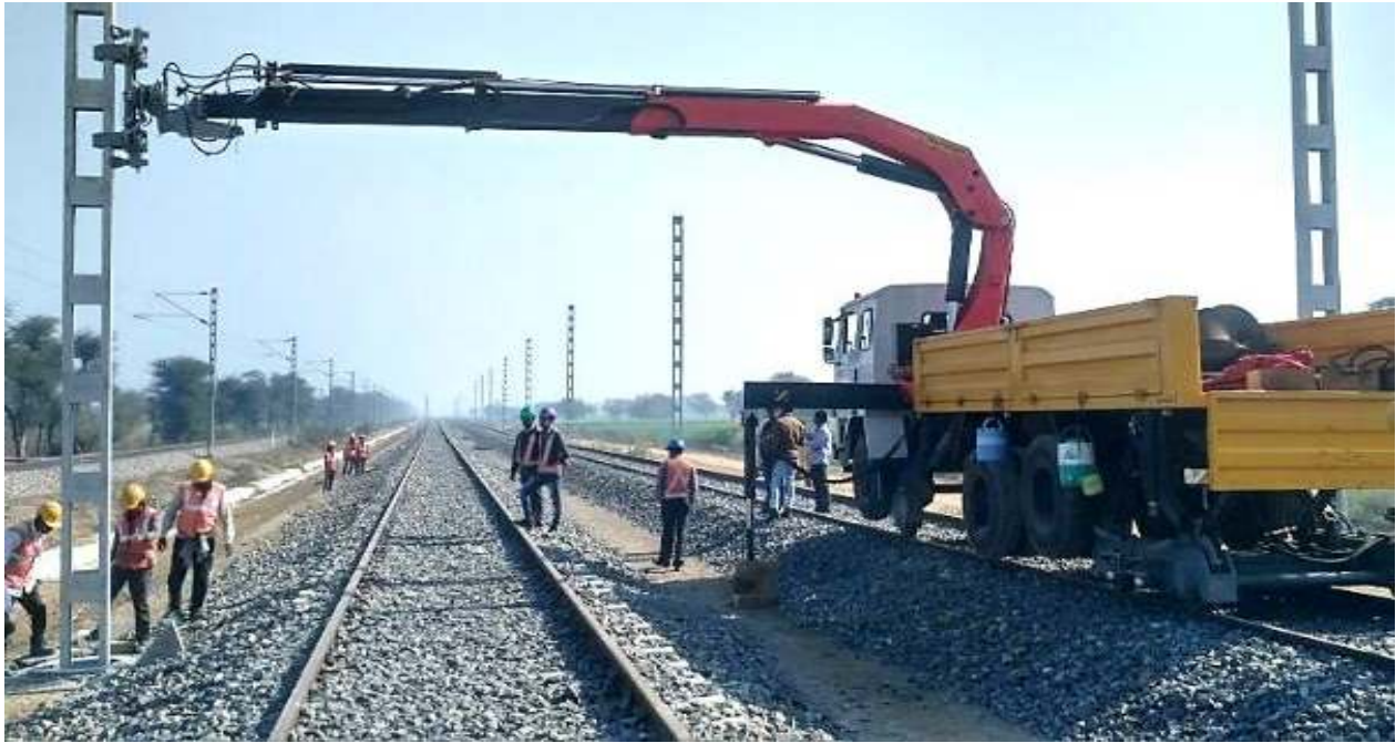
Fig. 9: RRV mounted Geismar mast grabber
