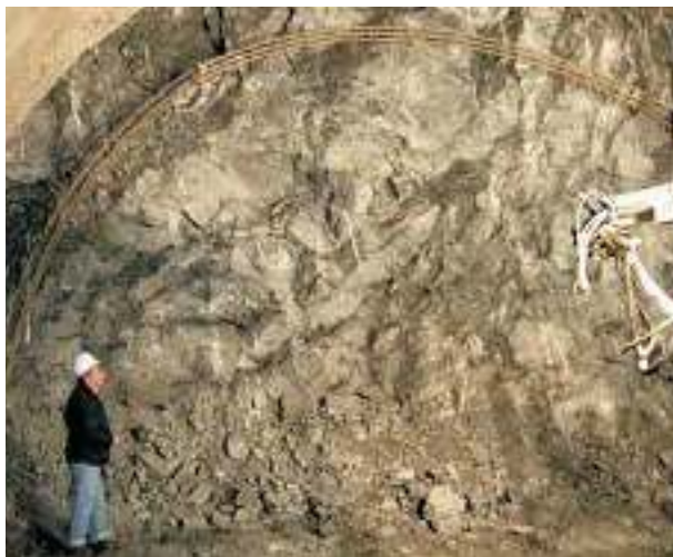
Fig-33 Steel Rib support at Portal-2(Dadri End)
