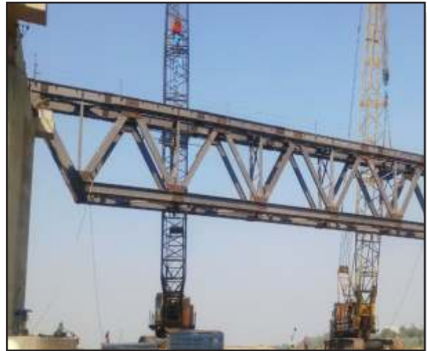
Launching of 8th Girder at Sabarmati Bridge
