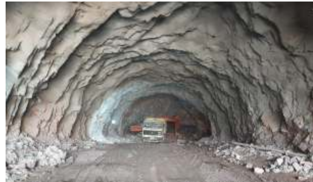
Fig-25 Mucking through Dumpers & Excavators
