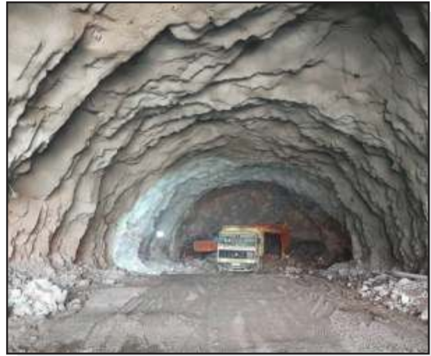
CTP-14 ,Mucking through Dumpers & Excavators in Tunnel
