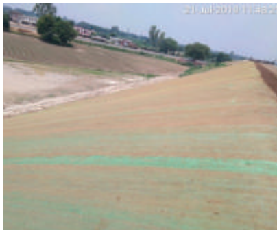
Fig. 7, 8, 9: Coir Mat Placement
