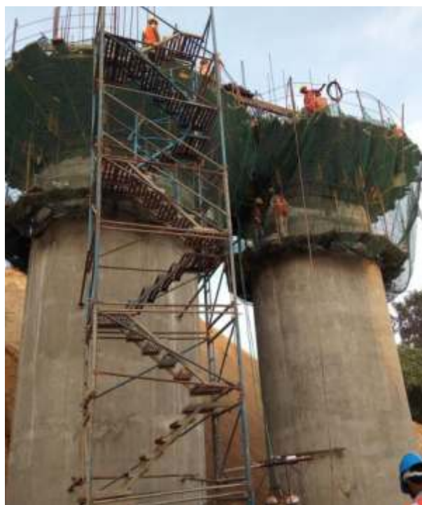
Fig. 5: Concreting using slip form
