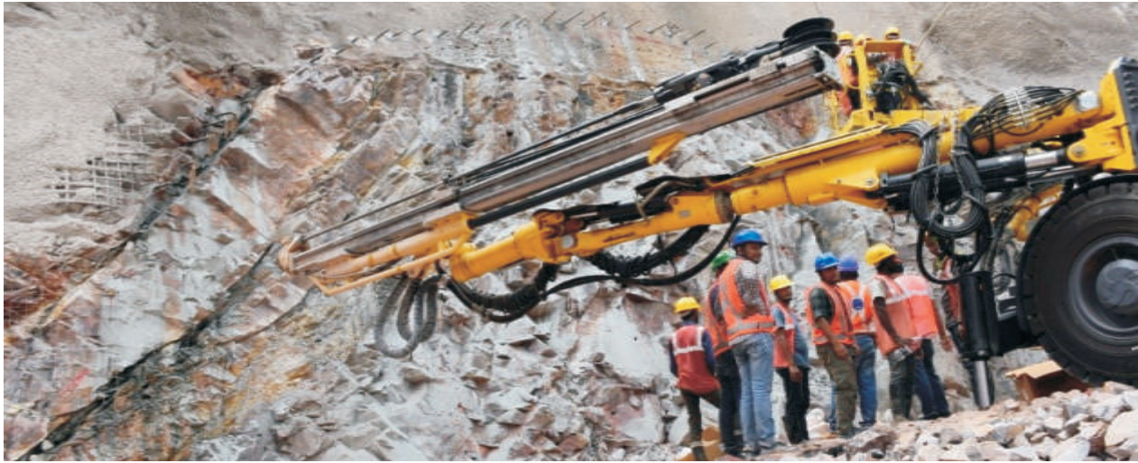
Fig-17 Site Photograph after Stage-III (for poling) of Portal Development
