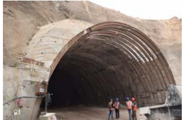
Fig-33 Steel Rib support at Portal-2(Dadri End)
