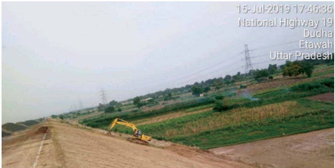
Fig. 6: Bed Preparation for Coir Mat
