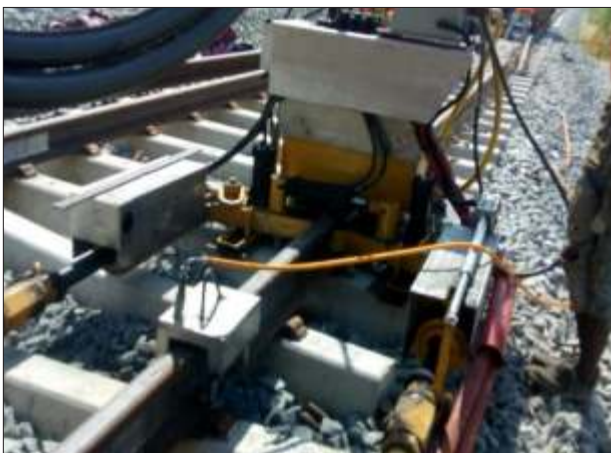
Fig. 7: Super puller machine for de-stressing
