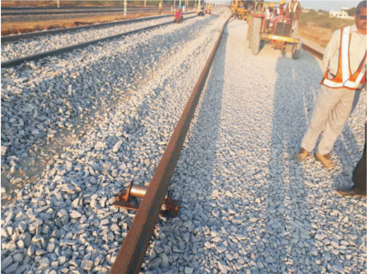
Pulling out rail panels
