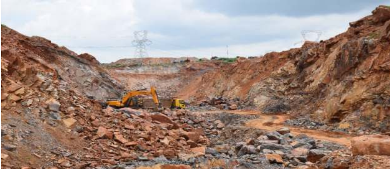
Figure-10 Excavation of approaches to reach the Portal Face Preparation for Portal
