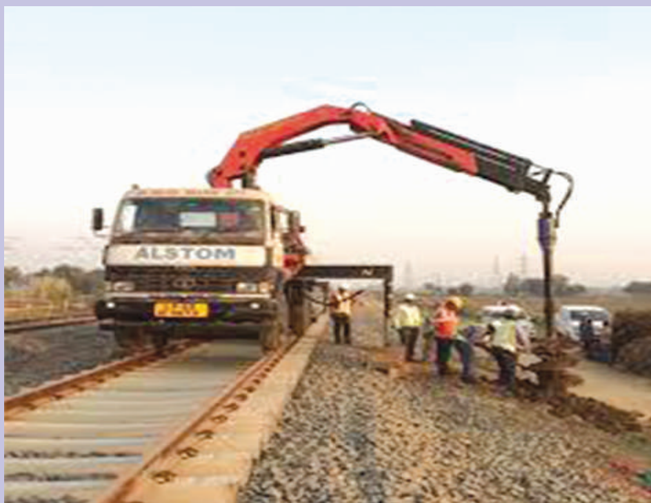
Fig. 8: Foundation Augring by RRV Colmar
