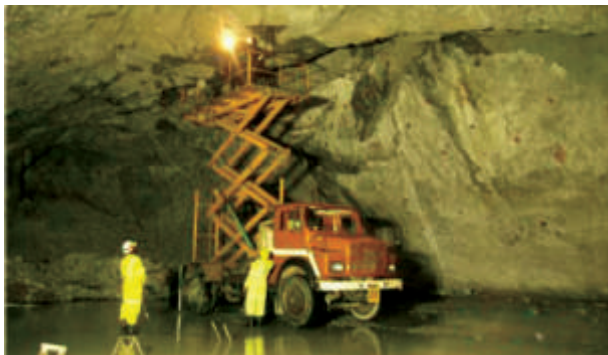
Scaling using Scissor Platform
