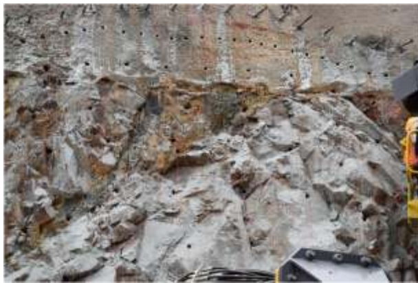
Fig-21 Photographs showing drilling & charging of holes at Tunnel face
