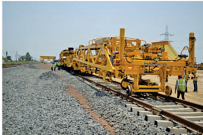
EDFC-1- Track linking NTC machine at Bhadan
