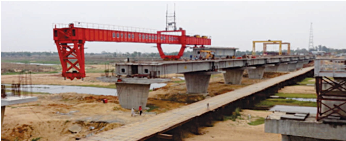
Sone-bridge - launching of girders
