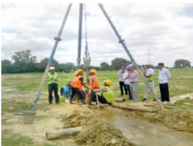
Geotechnical Investigation in Progress
