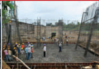
Bridge 359 on River Kaveri North in Western Corridor
