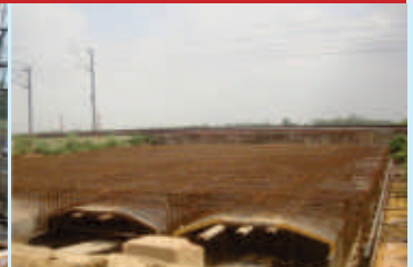
Bridghe No-662 in Eastern Corridor
