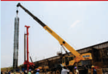
Bridge No-359 on River Kaveri North in Western Corridor
