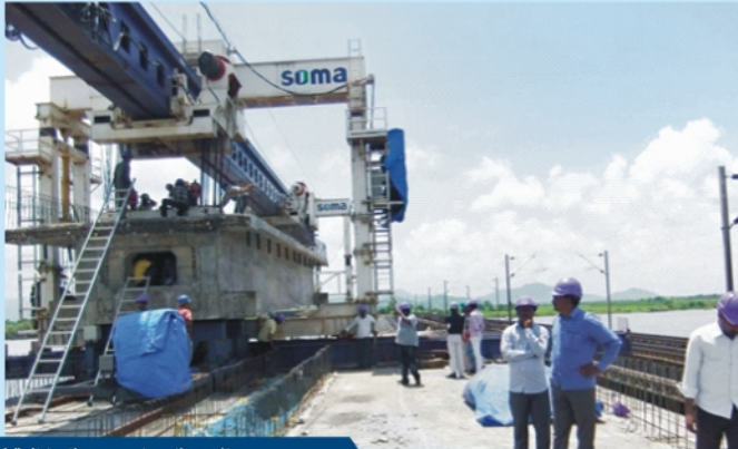
Visit to the construction site
