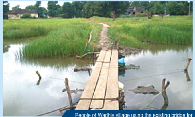
People of Wadhiv village using the existing bridge for daily commutation with main land
