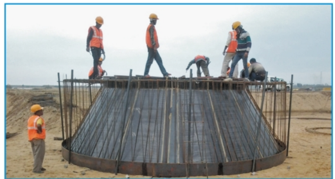
Construction of Sone Bridge started on EDFC.
