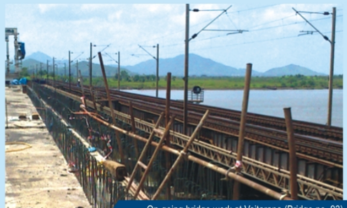
On-going bridge work at Vaitarana (Bridge no. 93)
