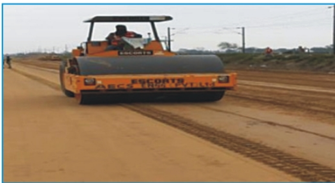
Construction started on Khurja-Bahupur section on EDFC at Aligarh.
