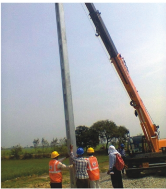
OHE Mast being erected
