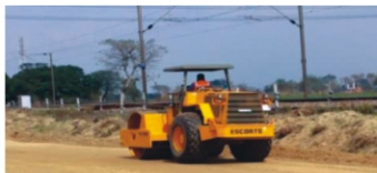
Preparation of Embankment Layers (CP 103) on Khurja-Bahupur section of EDFC (APL 1)
