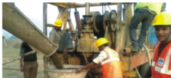
Concreting of Pile at Major Bridge No.304 on Khurja-Bahupur section EDFC (APL 1)
