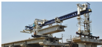
Launching of PSC Box Girder at P4-P5 of Bridge No. 359 at km 214/3-11 in Jorvasan-Bilimora block section between Bombay Central-Surat station in Valsad
