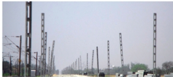
Erected OHE Masts in the section
