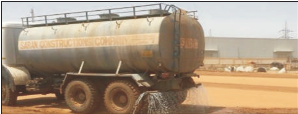
Fig 7: Watering of Soil
