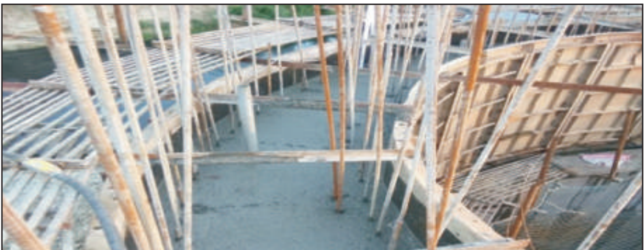
Upper view after concrete pour completion
