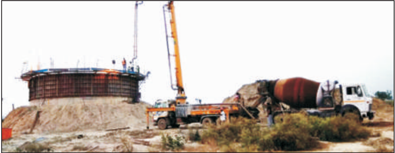
Concreting of well steining lift
