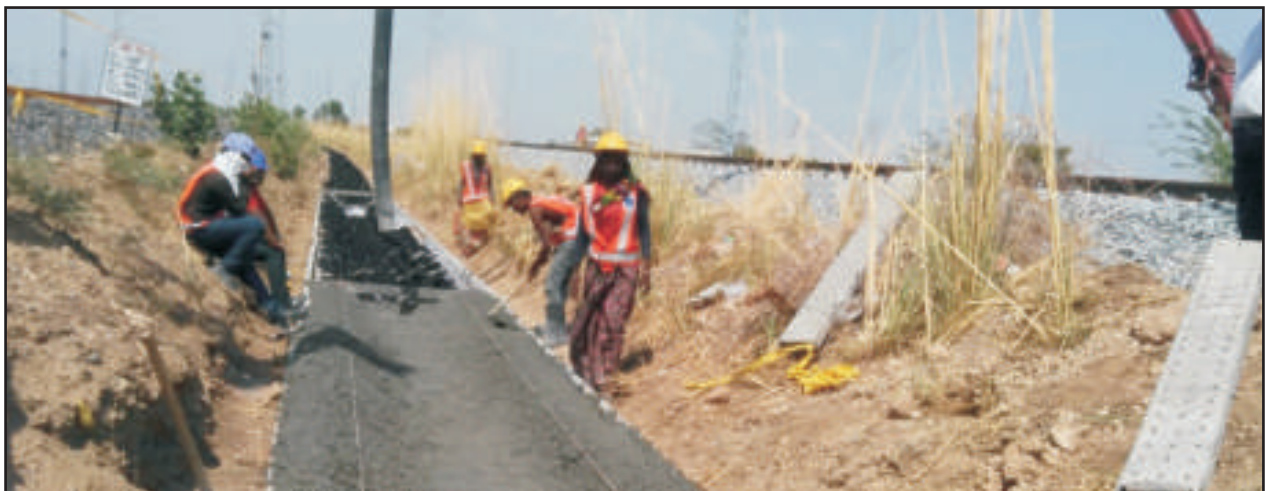
Concreting of Geocell drain
