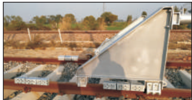
Figure -5: Frame of Friction Buffer Stop
