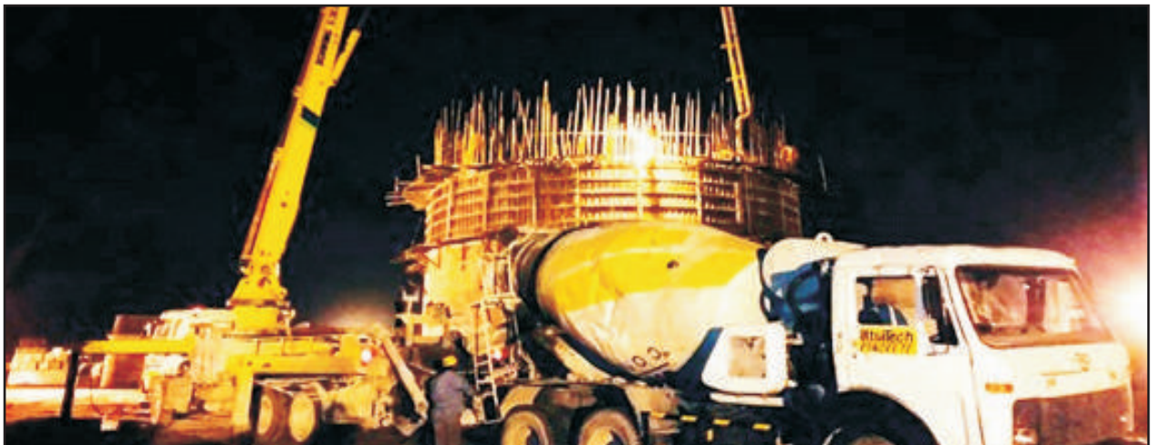
Concreting of well steining lift
