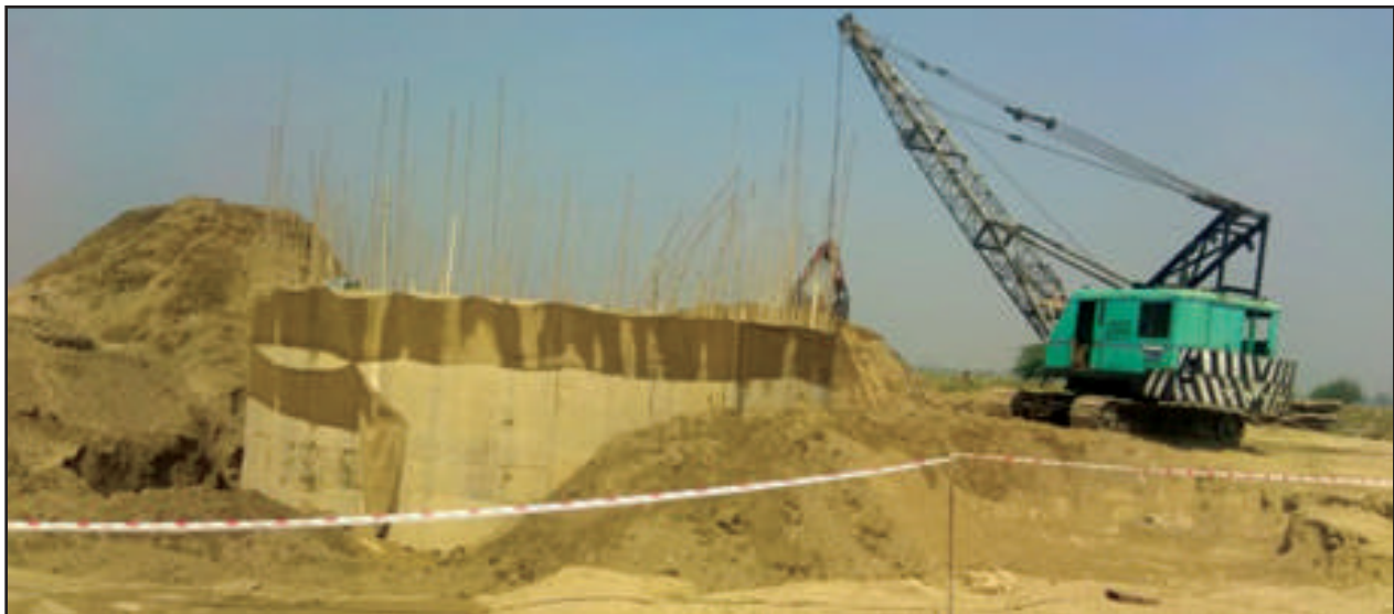
Curing of well steining lift in progress
