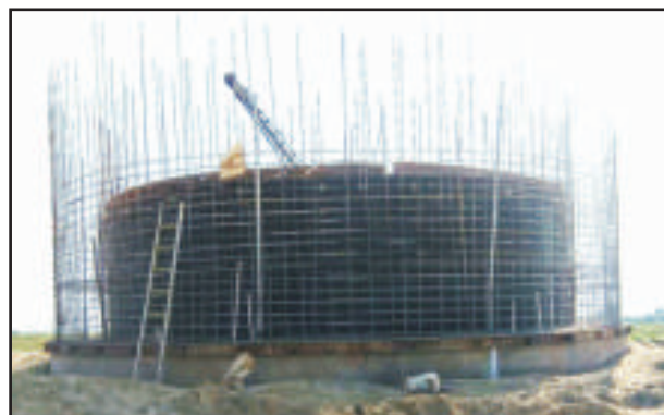
Fixing of inner shutter and rebar
