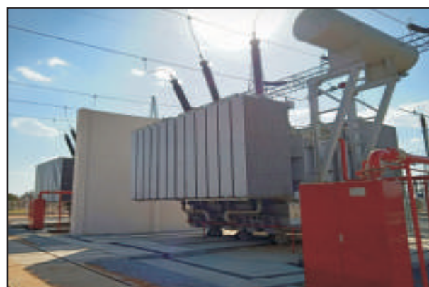
Fig.3. Scott connected transformers and NIFPS system at Ringus TSS
