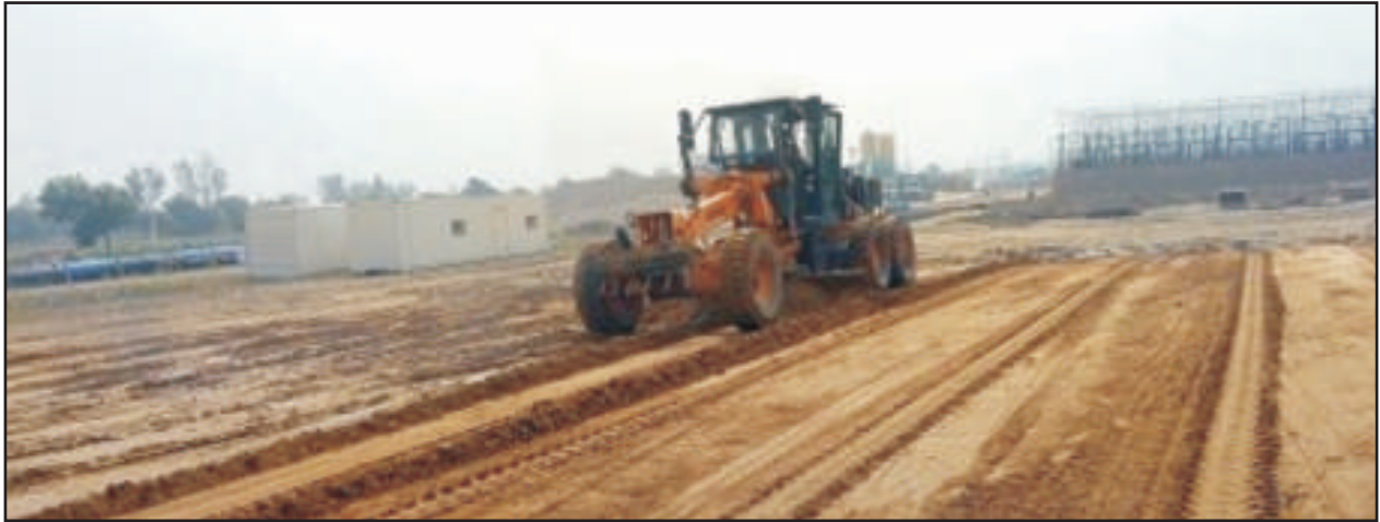
Fig 6: Spreading of Soil
