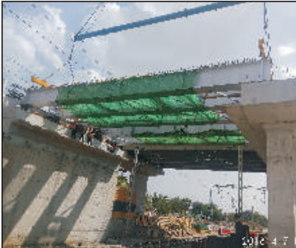
Steel girder launching on ROB at Ringus of WDFC section
