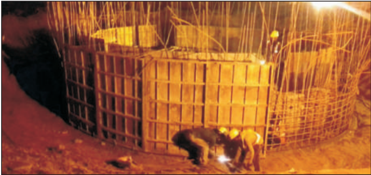
Fixing of the outer shutter
