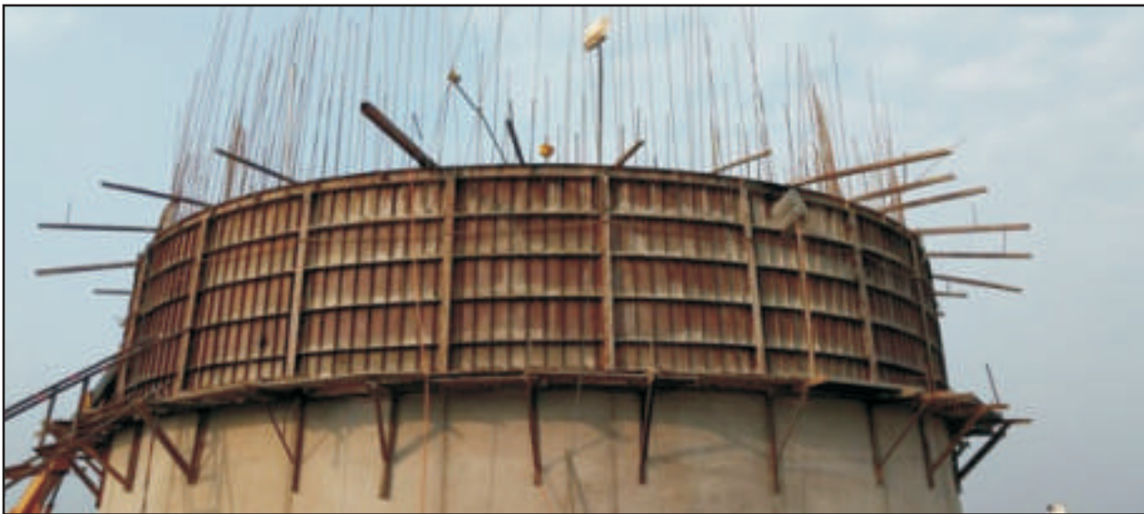
Complete fixing of the outer shutter
