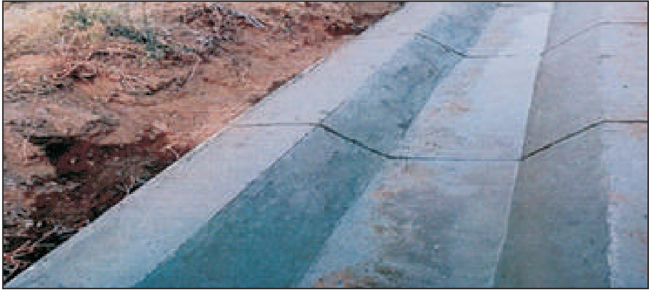
Finished Open drain constructed with Geocell
