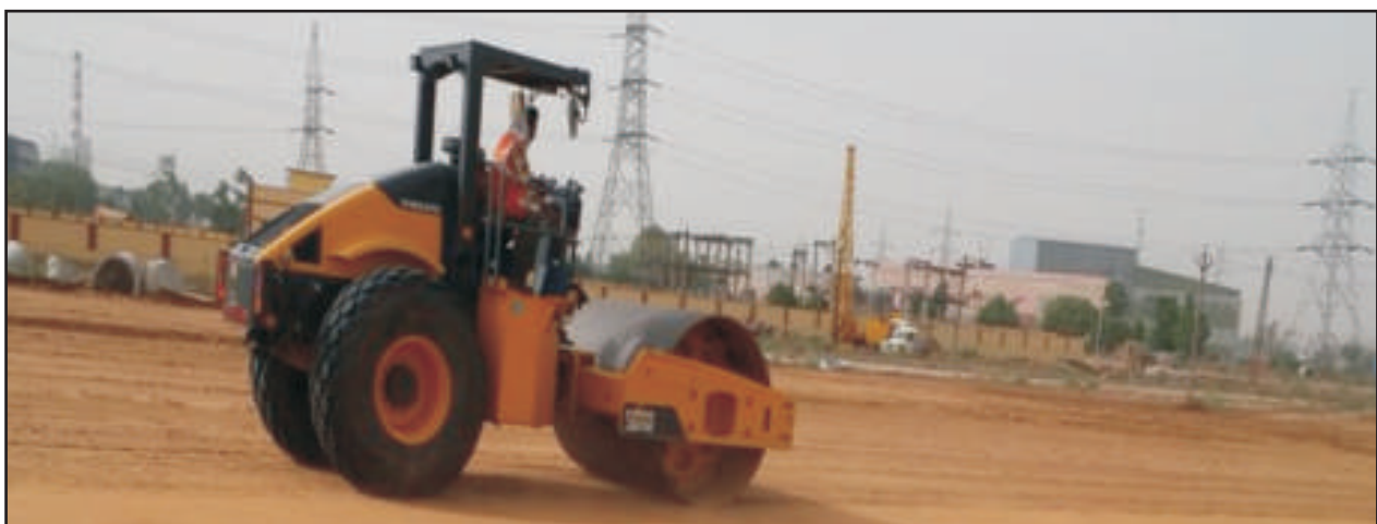
Fig 8: Rolling for Compaction of Soil
