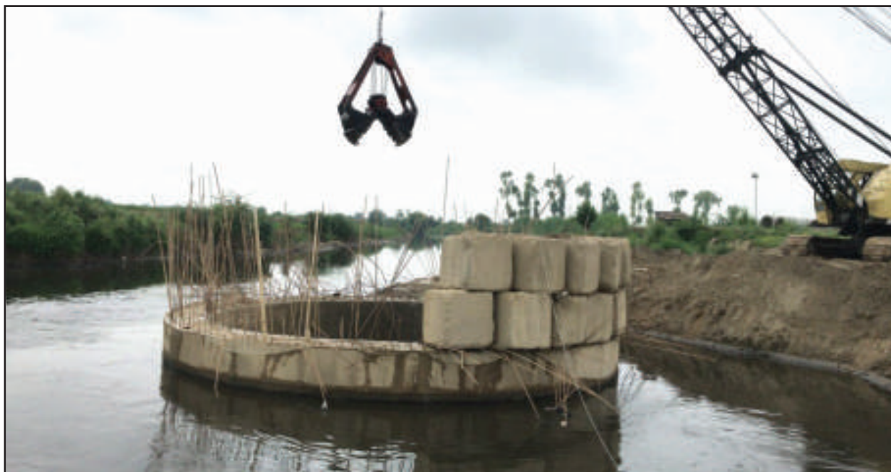
Eccentric loading to control tilt of well foundation
