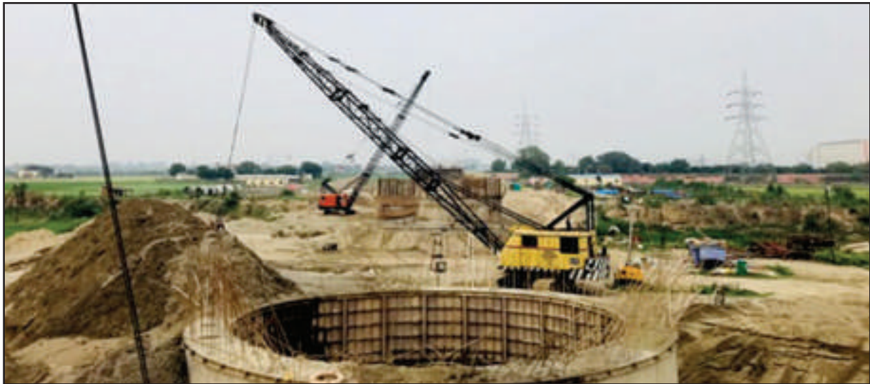
De-shuttering of the outer shutter
