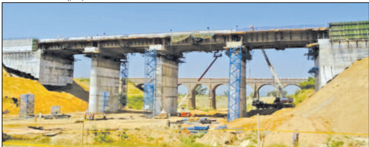
Construction of a major bridge at Maonda of WDFC section
