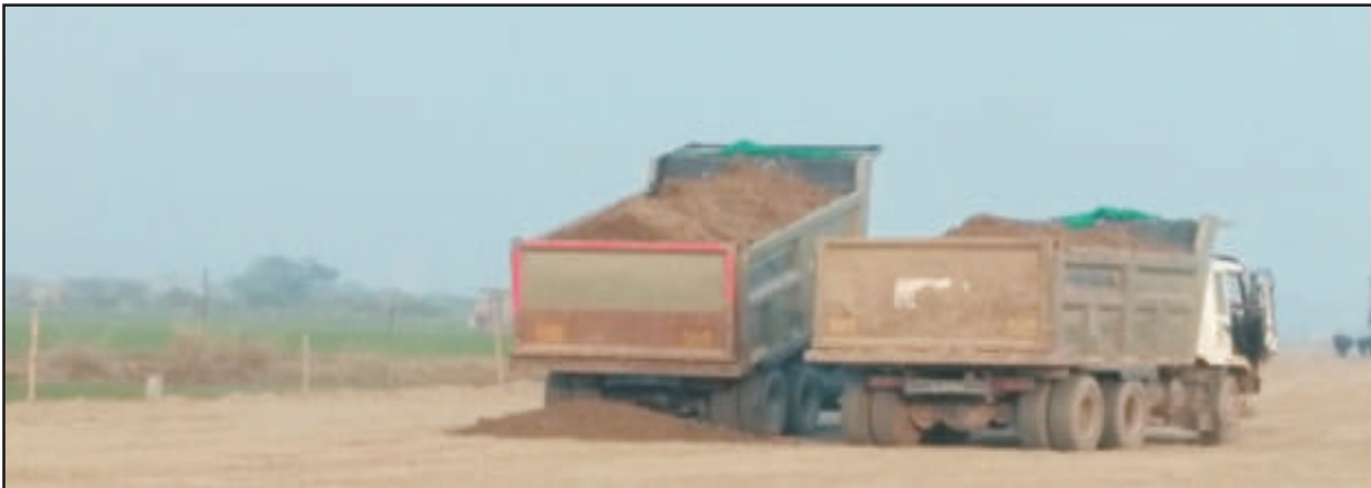
Fig 5: Dumping of Soil From Borrow Area
