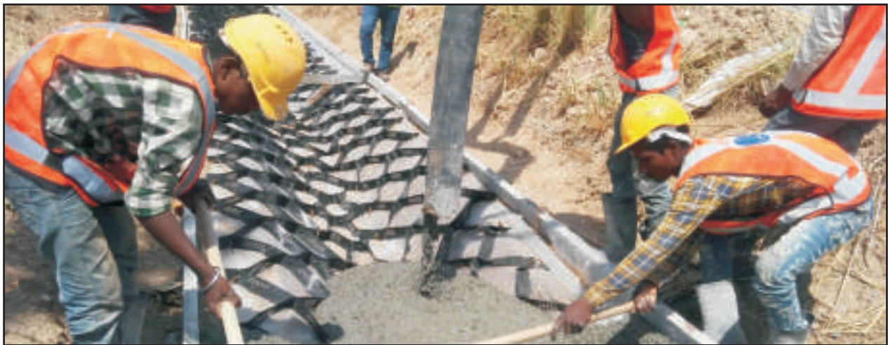
Finished Open drain constructed with Geocell
