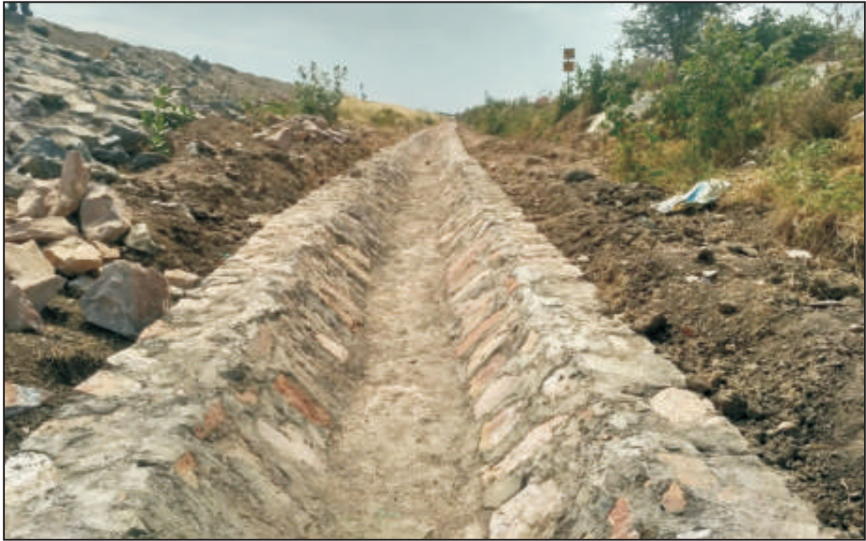
Stone Pitching Drain
