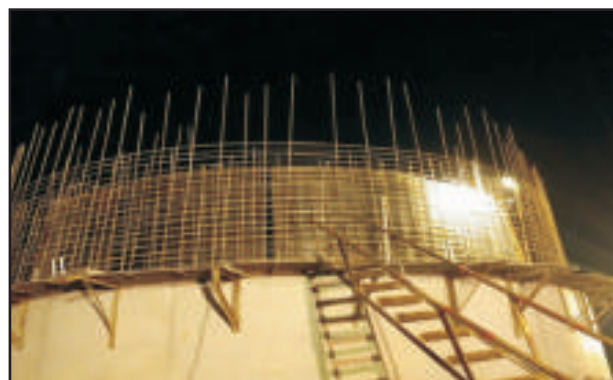
Fixing of rebar and access ladder
