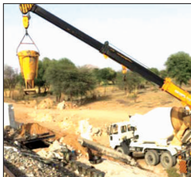
Crane bucket pouring method
