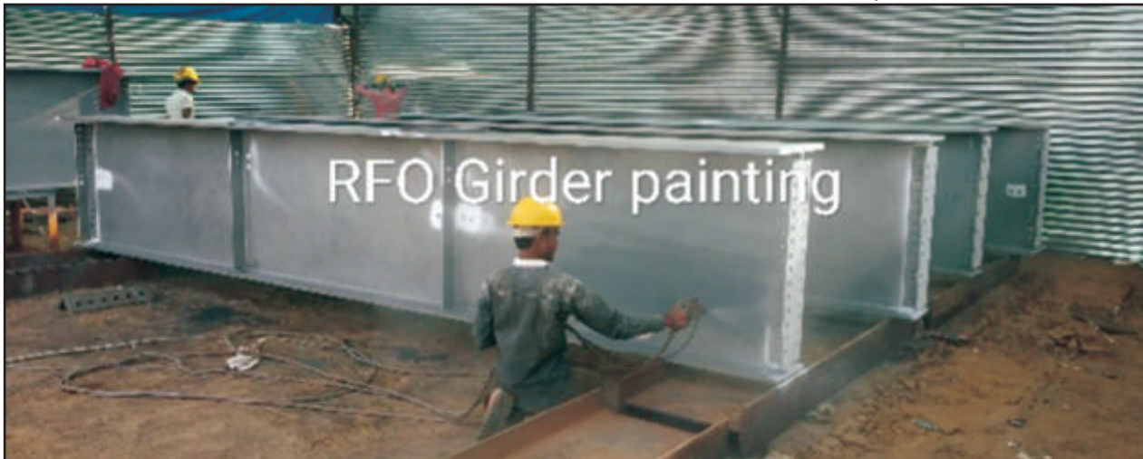
Painting of RFO Girder of Bridge no-136 in Rewari-Dadri Section of WDFC
