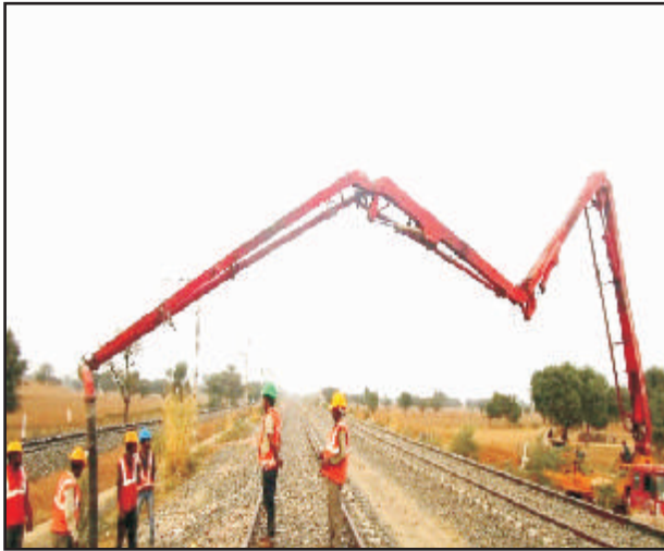
Fig.-7 Concrete pouring using boomplacer
