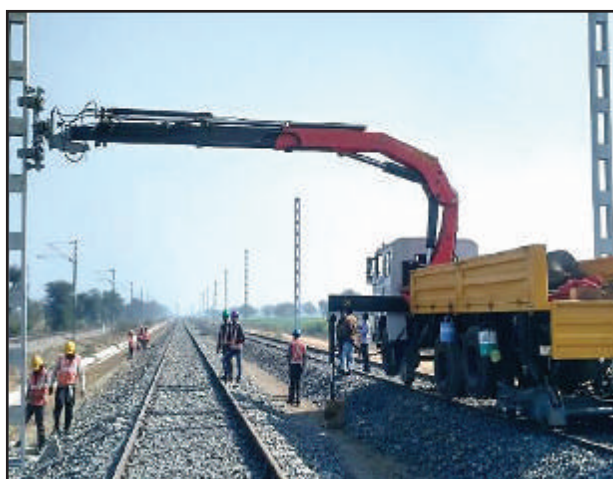
Mast grabber for mast erection, grouting and palfinger crane for mast erection
