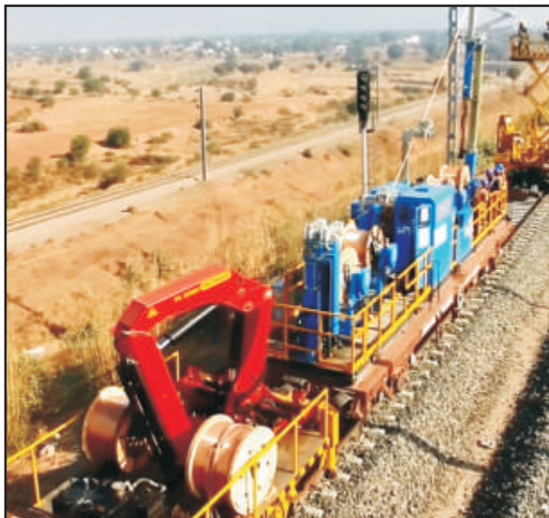
Fig.-10 OHE Wiring activity using wiring train
