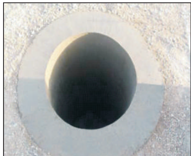
Finished cylindrical foundation
