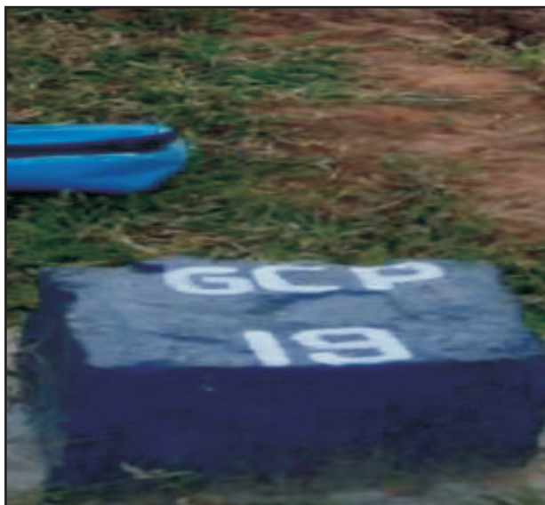
Fig.-9 Fixing of Bench Mark at 1Km. interval
