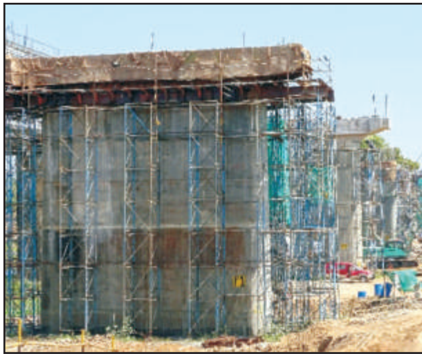
Curing of the Pier Cap of Bridge No. 19 over Damanganga
