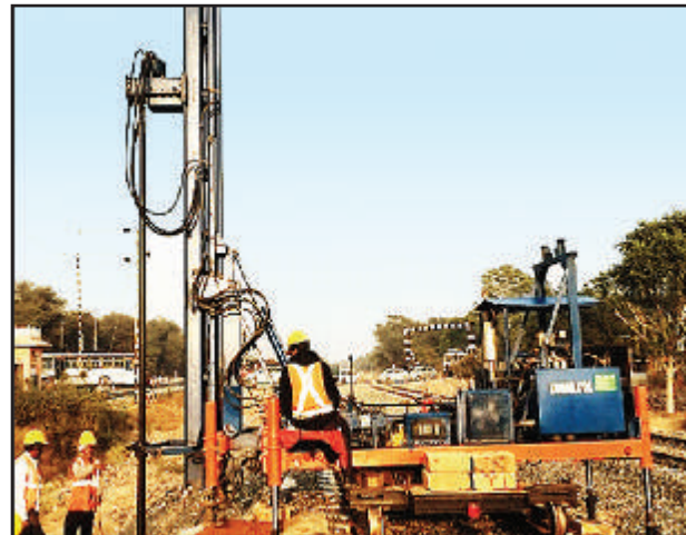
Fig.-2 Rail based augering equipment
