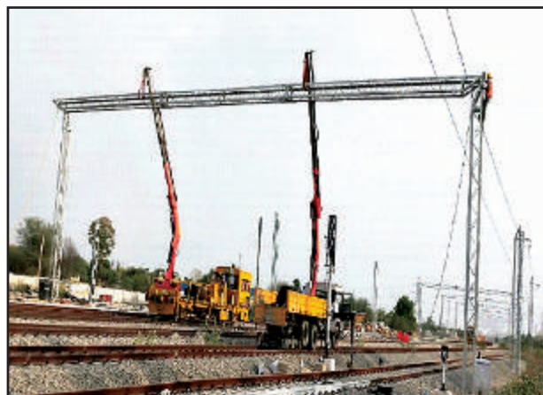
Boom erection using two Palfinger cranes
