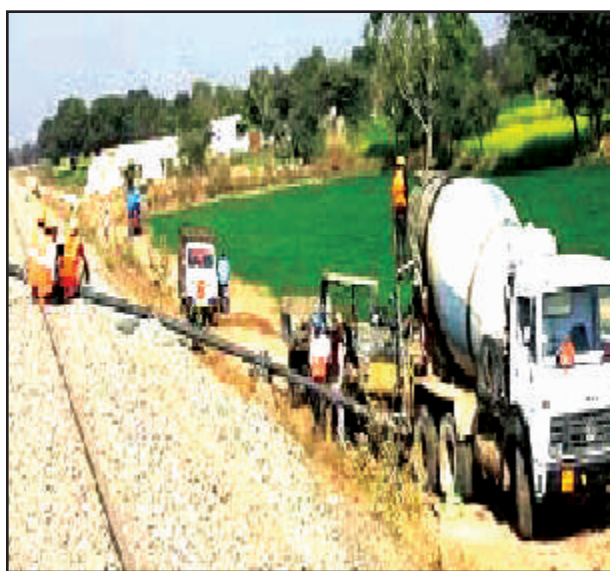
Concrete pumping through pipe
