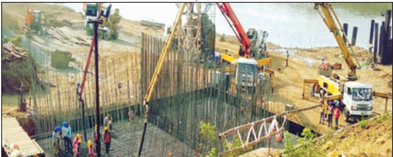
Concreting in progress for well cap of Abutment (A2) at Bridge No. 60 on River Par
