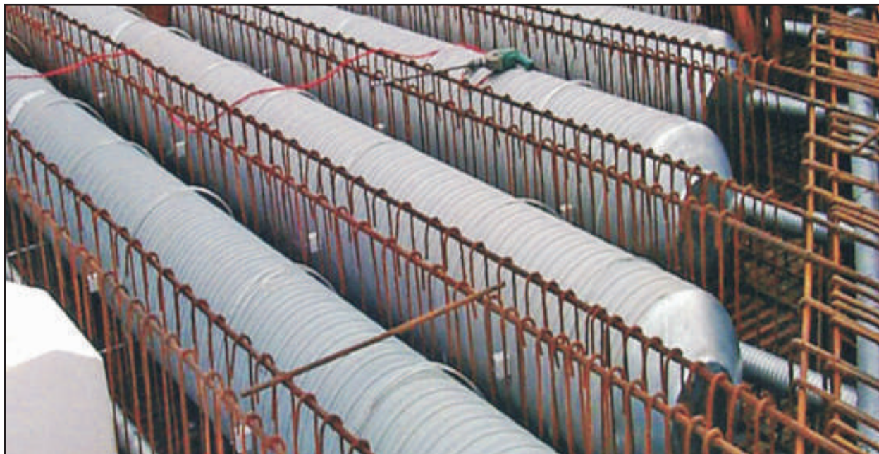
Figure 9: Tentative void former arrangement
