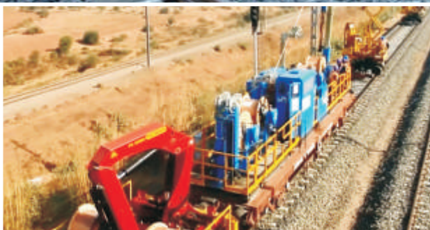
Pre-tamping survey using Survey trolley and Design Mode tamping using Absolute Profile on DFC Corridors
