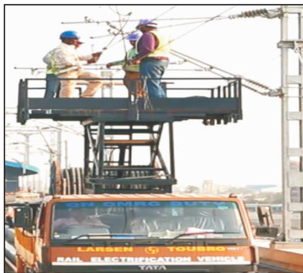
Fig.-14 Rail cum Road cantilever adjustment track
