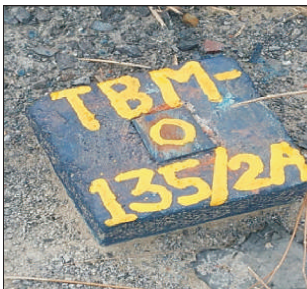
Fig.-10 Fixing of Temporary Bench Mark at 200m interval
