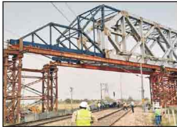
Fig-26: Second Stage Pulling of OWG
