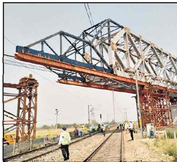
Fig-18: Cantilever pulling of OWG with the help of Launching Nose
