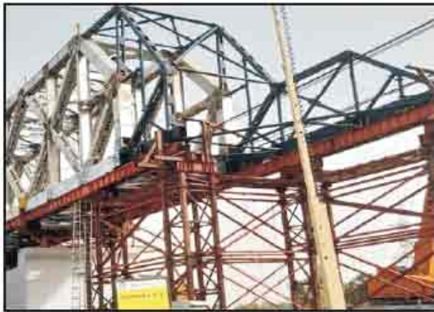
Fig-25: First Stage Pulling of OWG
