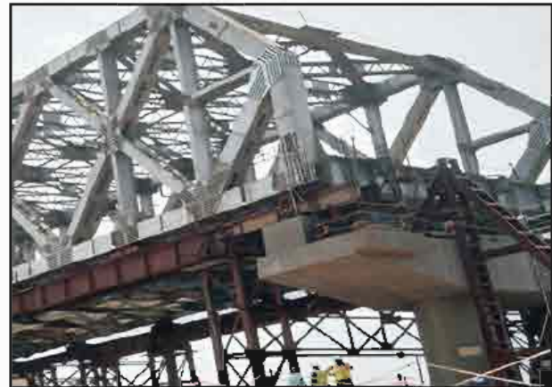
Fig-11: OWG after completion of Pulling
