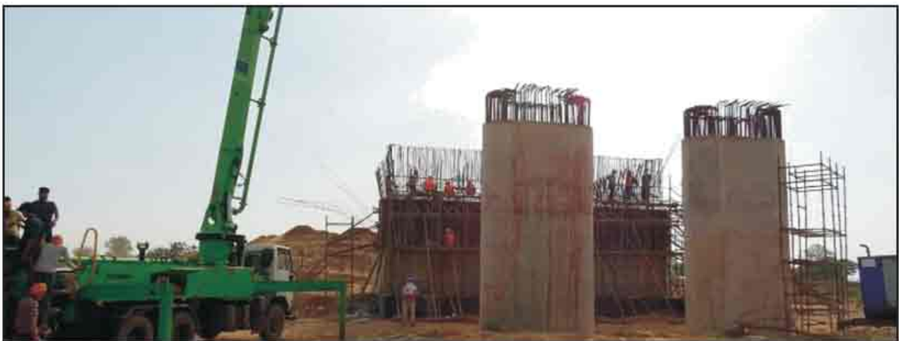
Concreting in progress (2nd lift) at Abutment (A1) of Bridge no. 69 of WDFC
