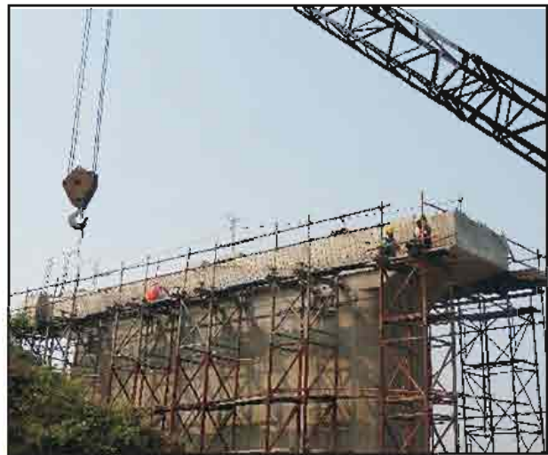
P1 Bearing inspection plate form work in Progress at Br. No. 240 Tapi
