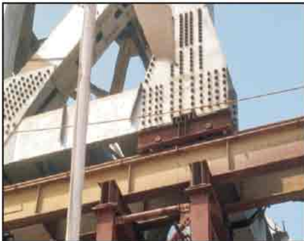
Fig-8: Movement of OWG supported on 4 Wheeled Trolley
