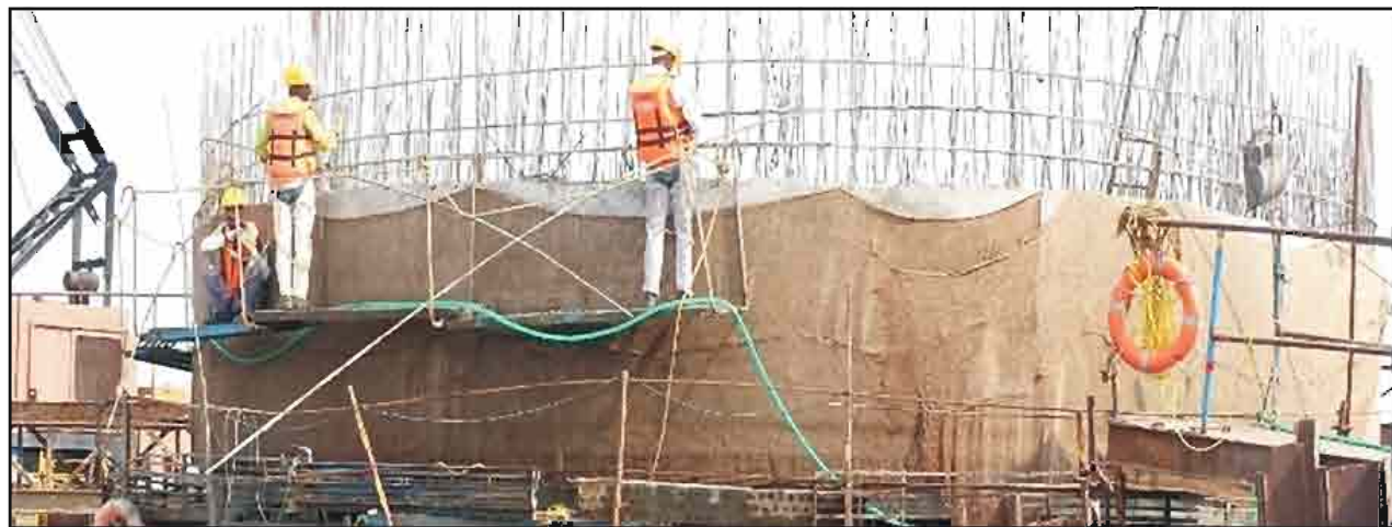
Final lift reinforcement for well steining of Pier P-12 in progress at Narmada Br. No. 57
