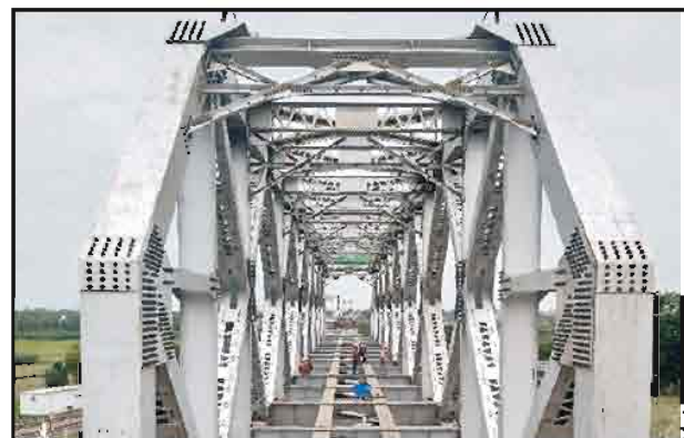
Fig 1: Open Web Girder (OWG)
