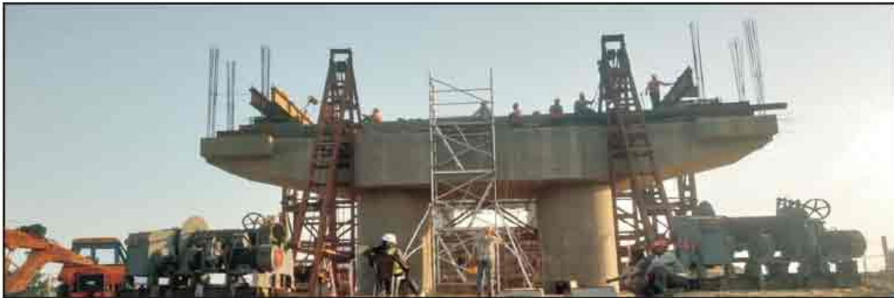
Fig-6: Installation of Winch Machine & Vertical Frame
