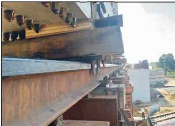
Fig-12: PTFE Sliding Block
