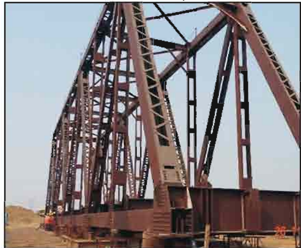
2nd Stage HSFG Bolt Tightening in Progress for Down Track Side Girder at RFO Site
