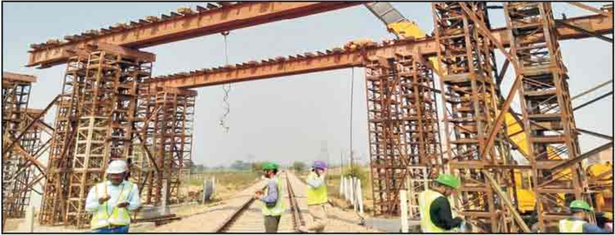
Fig-13: Temporary Staging
