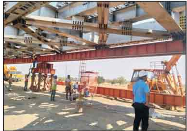
Fig-21: Launching Beam fitting under Bottom Chord
