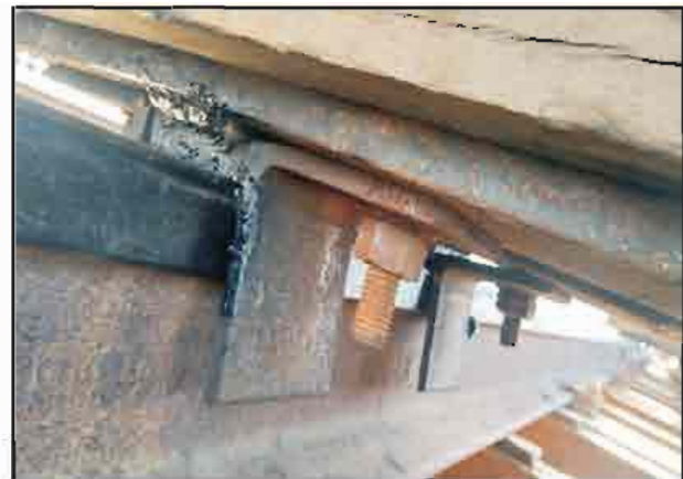
Fig-12: PTFE Sliding Block
