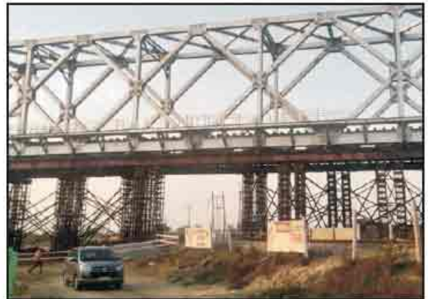
Fig-17: OWG after completion of pulling
