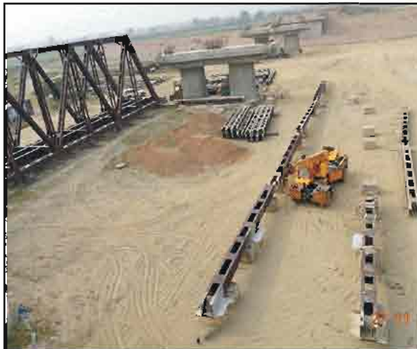
Main Assembling B/w P2-P3 Piers and Bottom Chord Assembling in Progress at Yamuna Bridge
