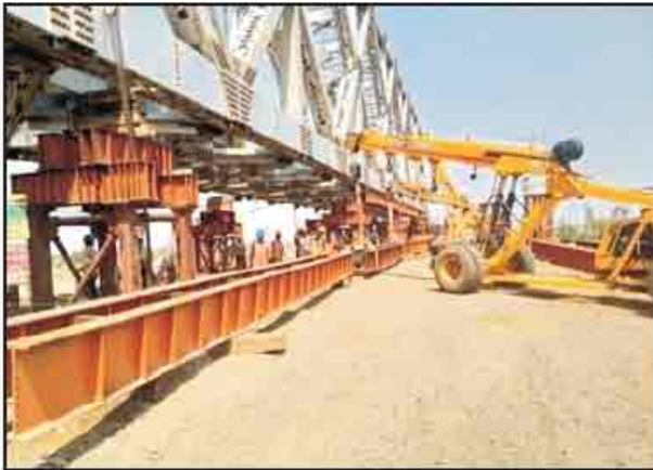
Fig-21: Launching Beam fitting under Bottom Chord
