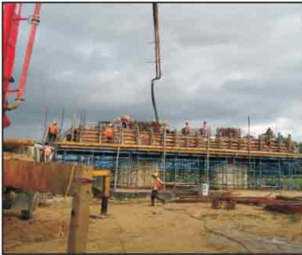
Concreting of pier Cap P2 at Br. No. 141 (CTP-14)
