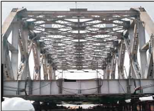
Fig-10: Pulley & Wire Rope Connected to OWG in pulling
