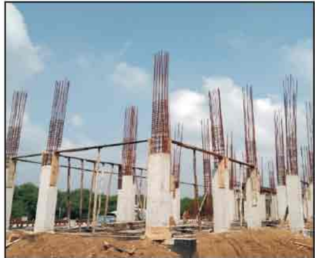
1st lift of Column completed & Beam Shuttering in progress (Ancheli Station Building)
