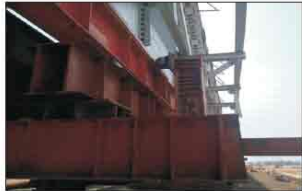
Fig-23: Lateral Guide Roller
