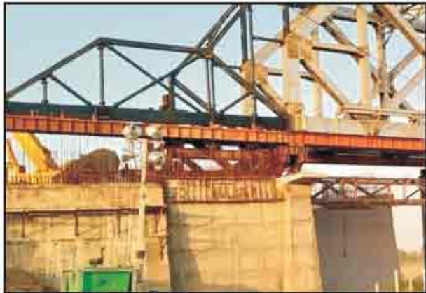
Fig-27: Third Stage/Final Pulling of OWG
