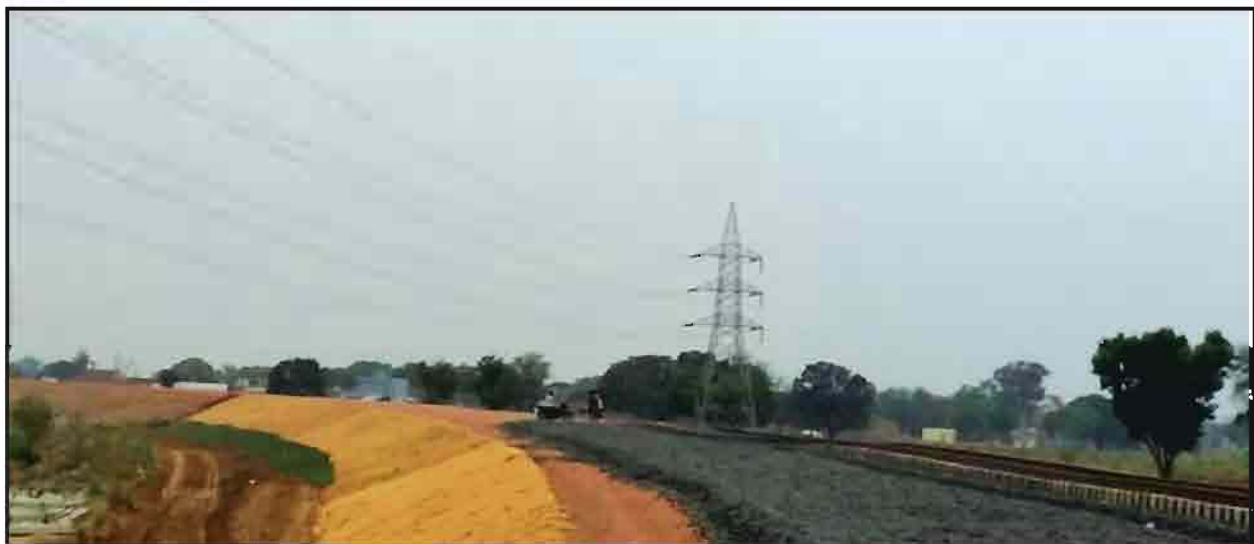
132 KV Transmission Line tower infringing DFC Track
