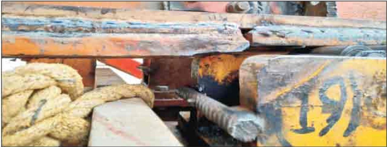
Fig-28: Bottom Flange of Launching Beam trapped by Collar of Hillman Roller
