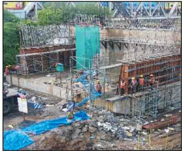
Abutment (A1) pedestal casting completed at PAR Br. No. 60 (CTP 15A)
