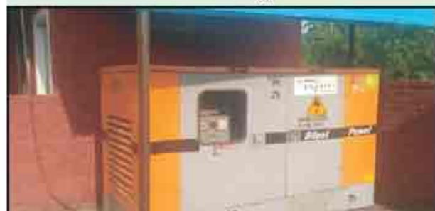
62.5 kVA DG set to supply of electricity
