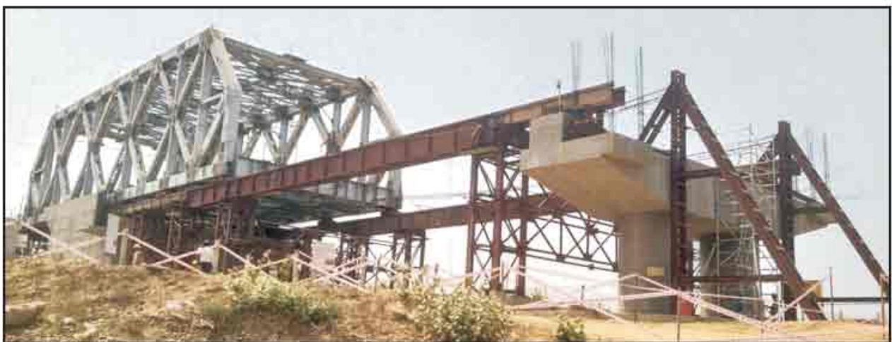
Fig-9: Pulling of OWG in progress showing the vertical frames
