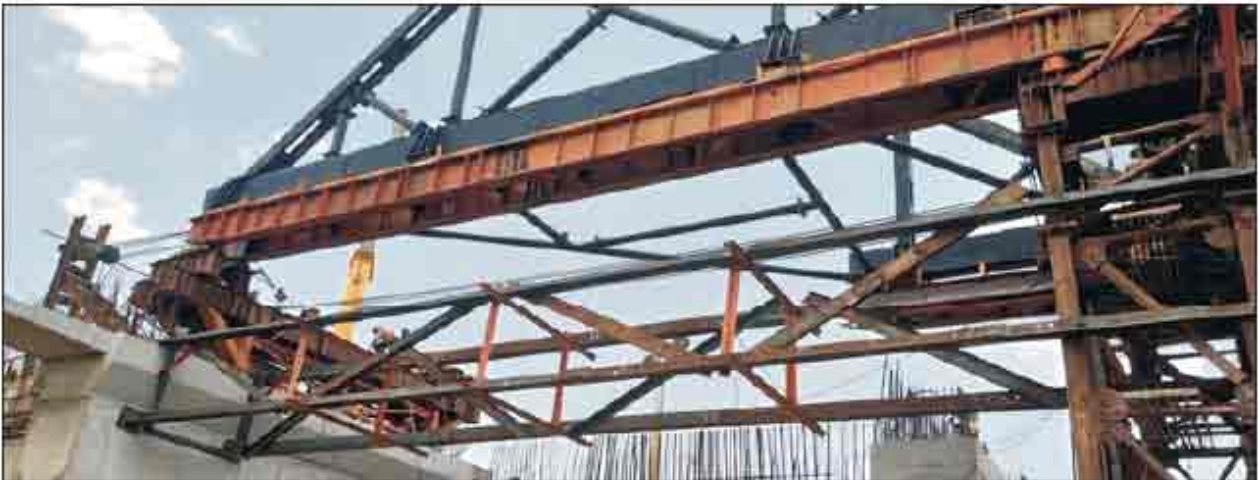
Fig-29: Reaction Truss erected to support the trestle
