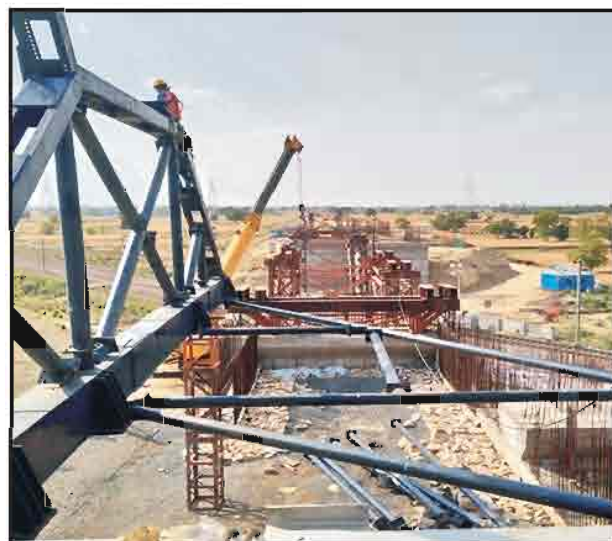
Fig-19: Launching Nose
