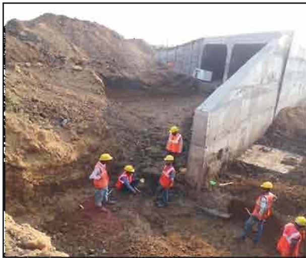
RCC Toe Wall in progress at Minor Bridge No. 147 of WDPC
