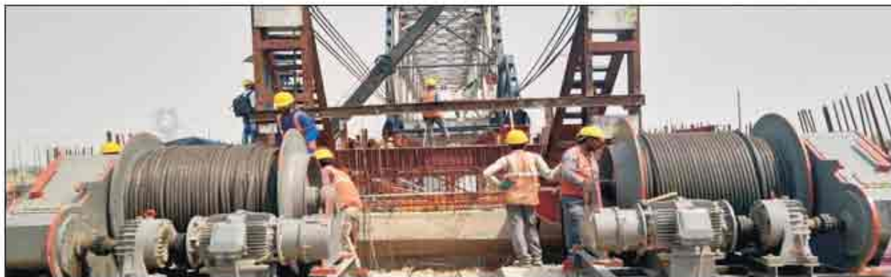
Fig-24: Pulling Mechanism
