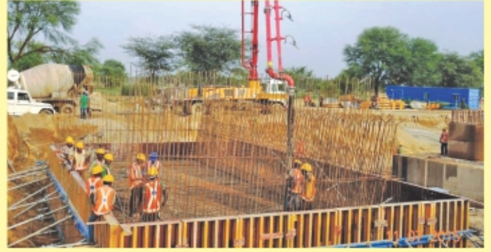
WDFC- Concreting of Pile Cap at Major Bridge in progress
