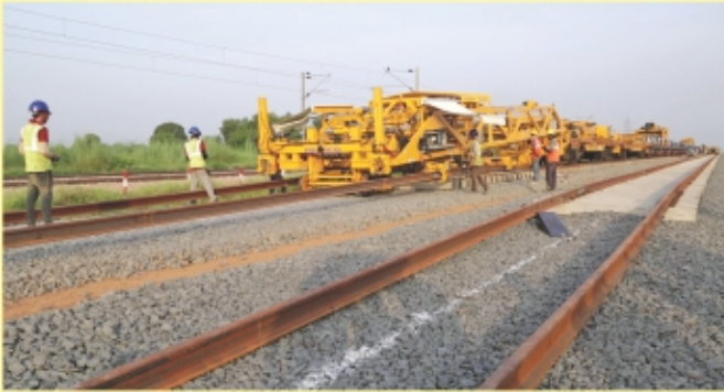
Laying of tracks with NTC machine at Bhadan on New Bhaupur-Khurja Section
