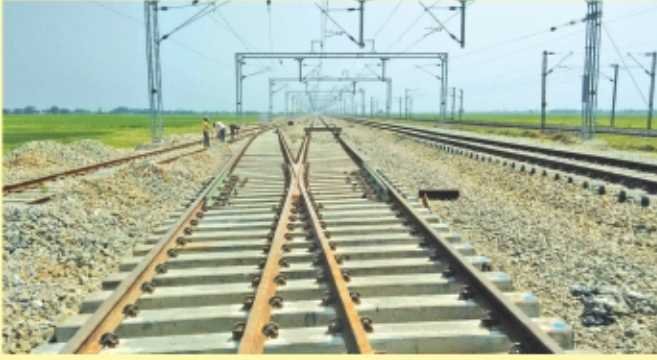
Canted turnout laid at Dugawati
