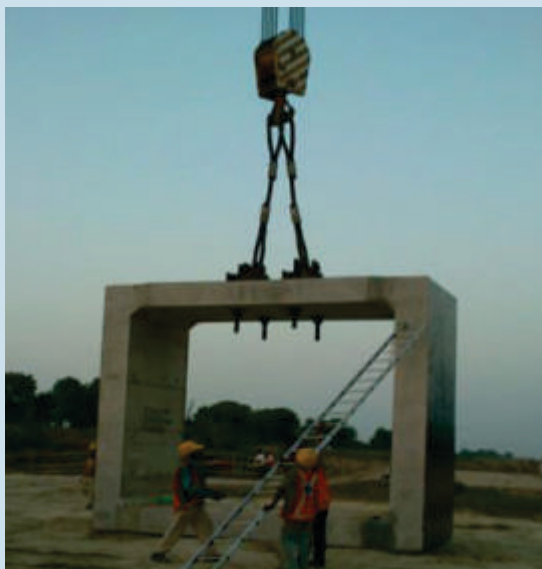
Precast segment staking, transportation and erection
