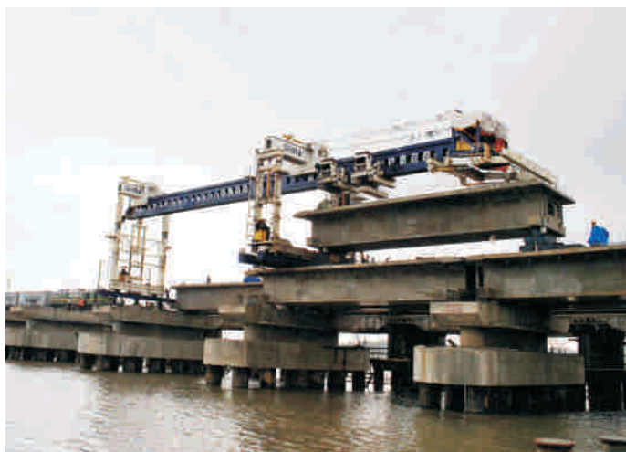
Launching of PSC Box Girder at P 17-P 18 of Bridge No. 93, at km 70/12-26 in Vaitarna-Saphale block section between Bombay Central-Surat station in Thane District of Maharashtra
