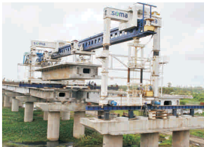
Launching of PSC Box Girder at P 3-P of Bridge No. 400, at km 238/5-11 in Navsari-Maroli block section between Bombay Central-Surat station in Navsari District of Gujarat
