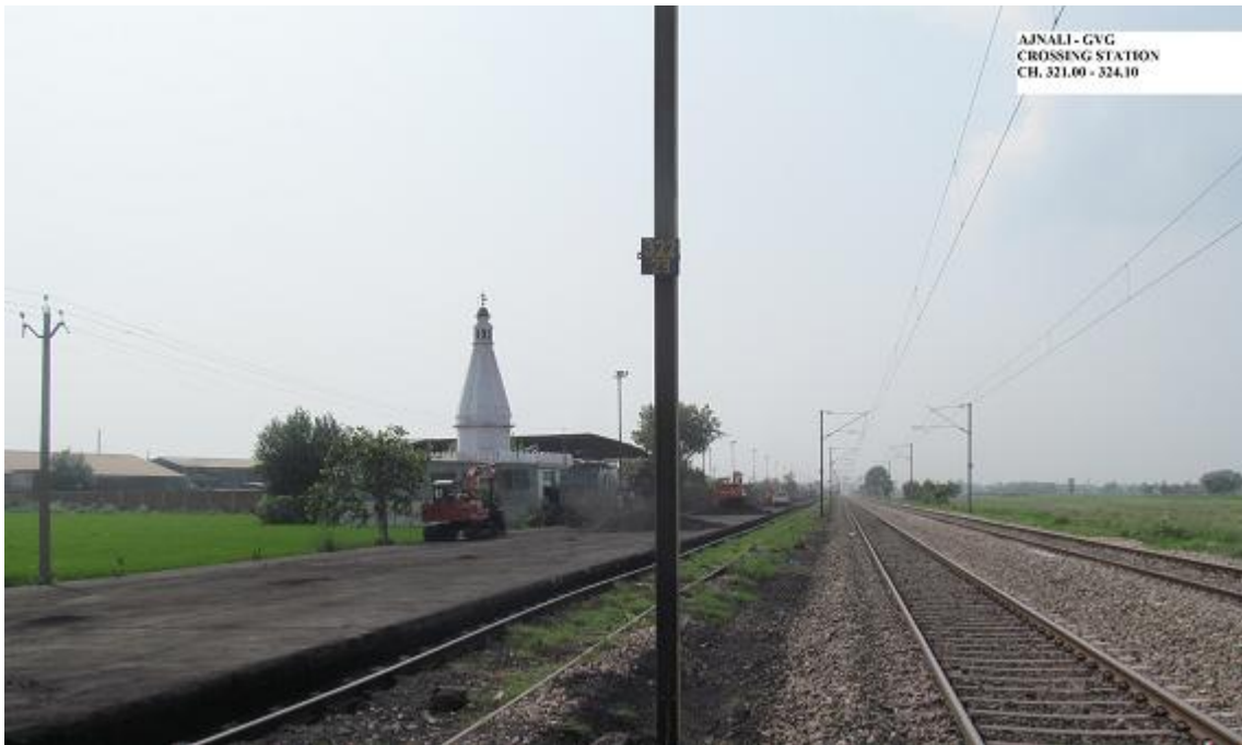
Figure 2.15 : Site for New Govindgarh Crossing Station
