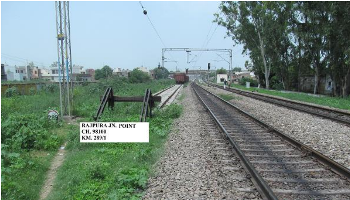
Figure 2.10: Location of Rajpura Junction Point
