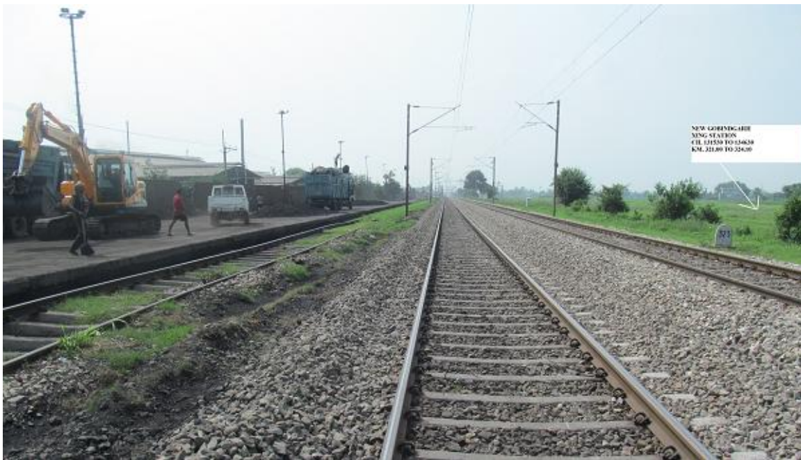
Figure 2.9 : Site for New Govindgarh Crossing Station
