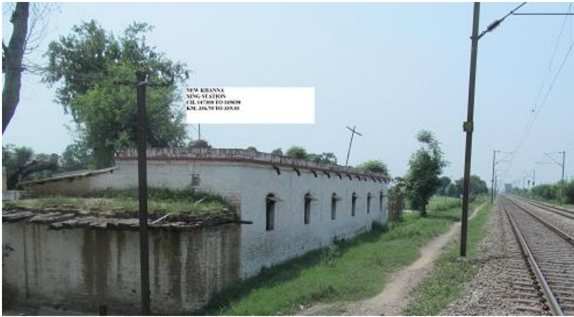
Figure 2.8: Site for New Khanna Crossing Station
