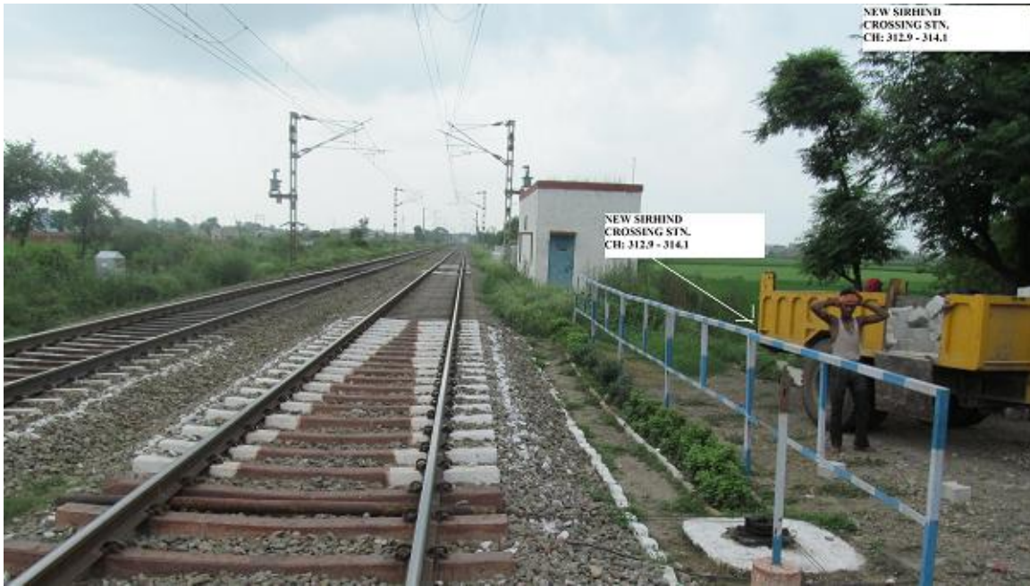
Figure 2.14 : Site for New Sirhind Crossing Station
