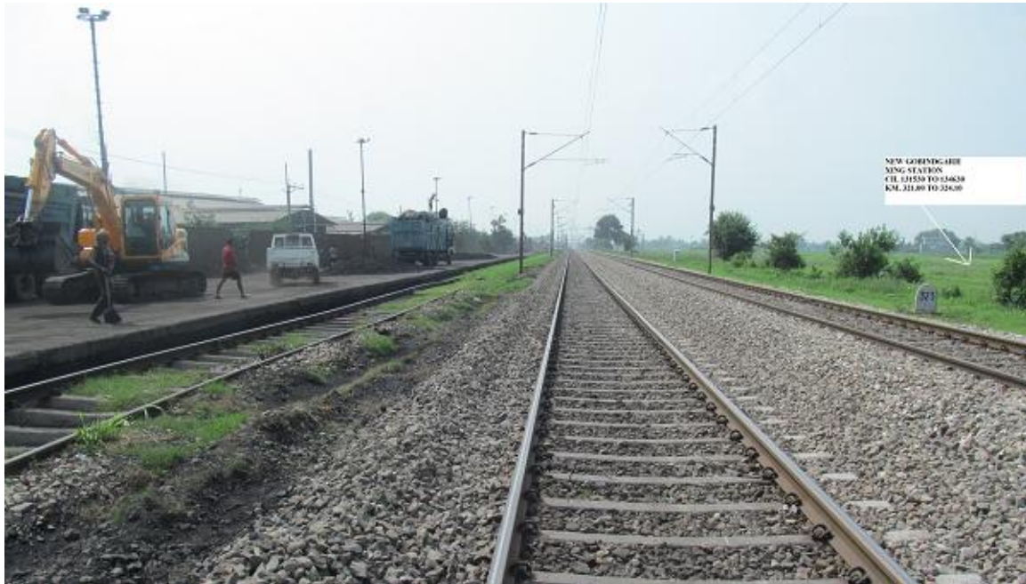
Figure 2.9 : Site for New Govindgarh Crossing Station
