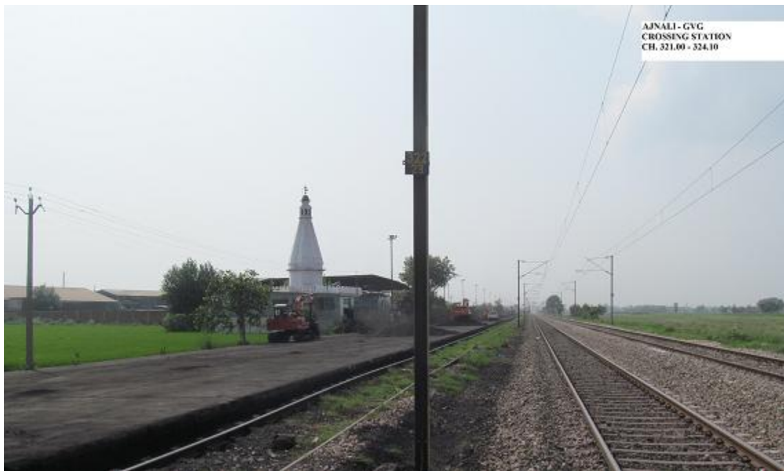
Figure 2.15 : Site for New Govindgarh Crossing Station
