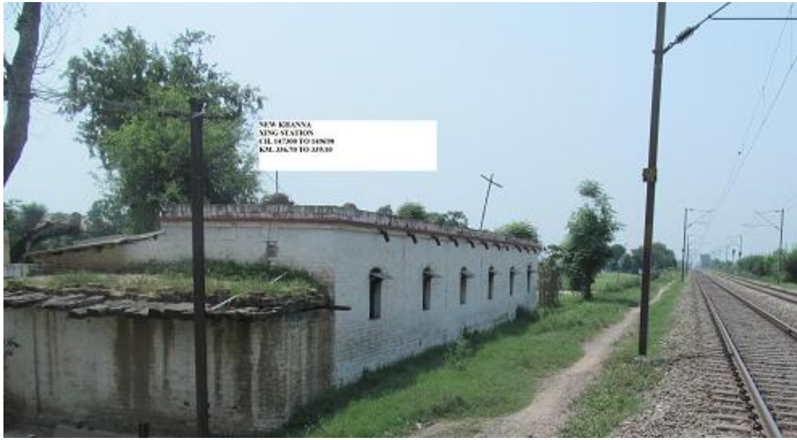
Figure 2.8 Site for New Khanna Crossing Station
