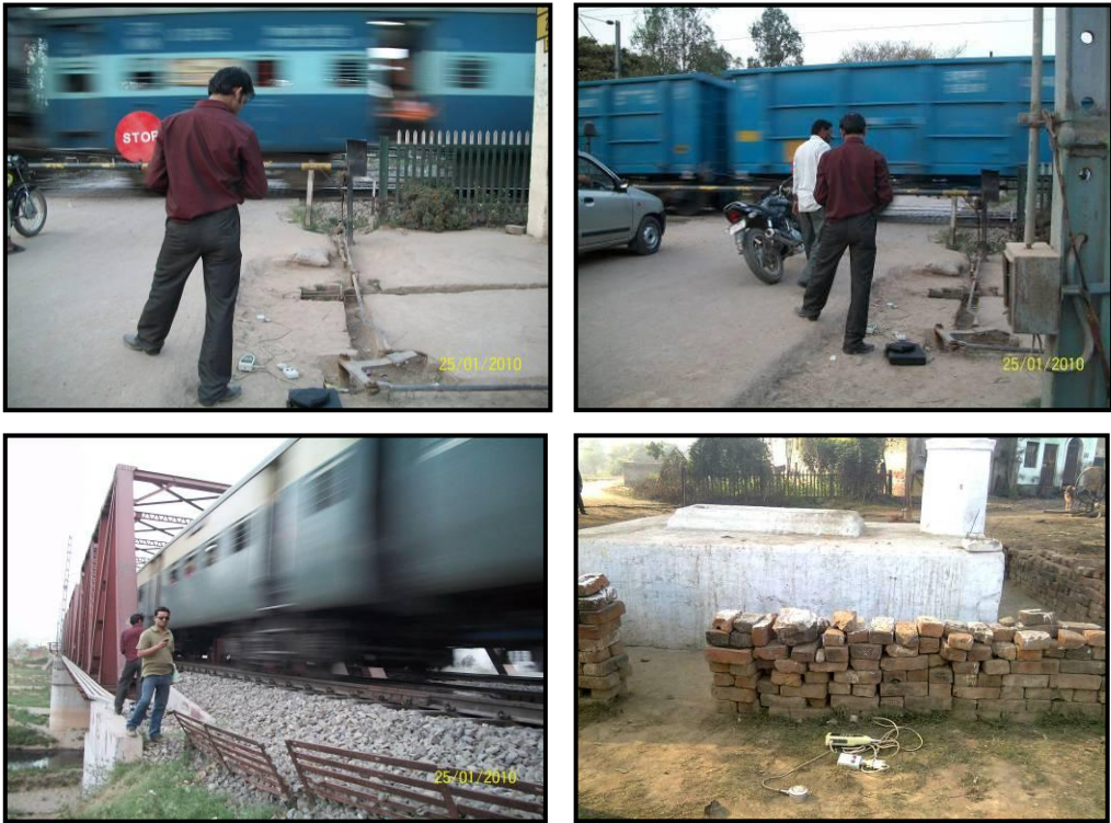
Vibration Monitoring Along the Alignment
