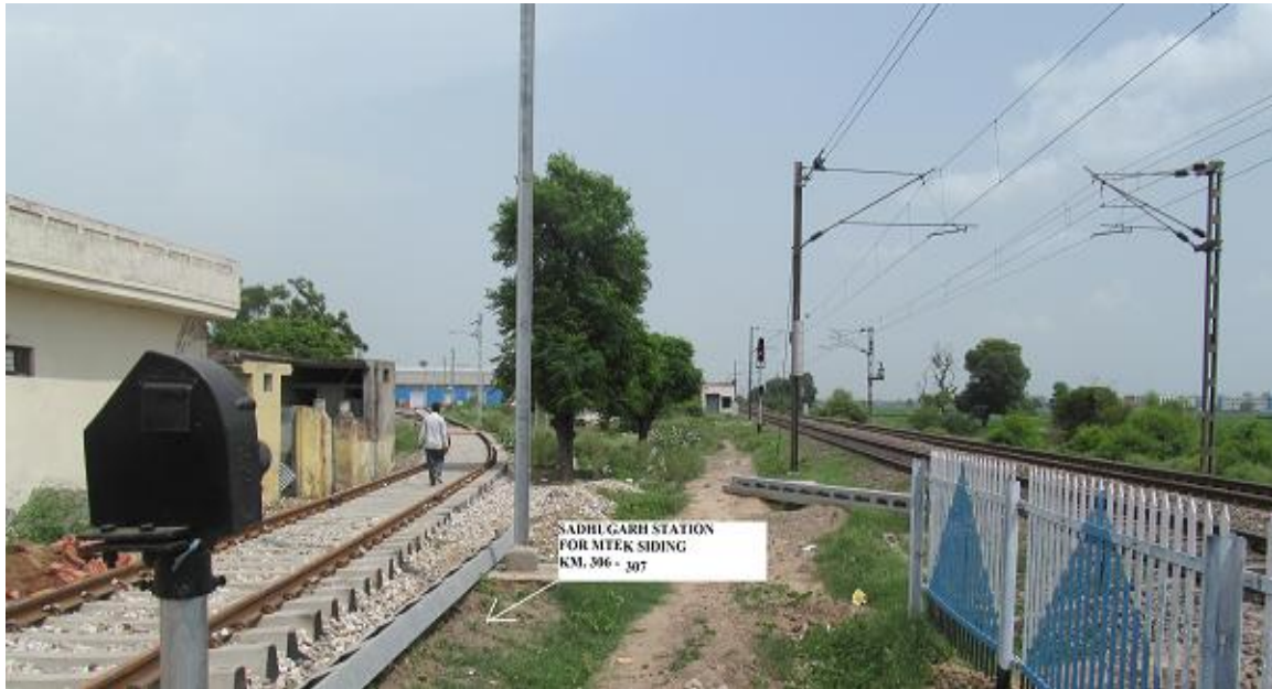
Figure 2.13 : Site for Proposed Sadhugarh Station and MTEK Siding
