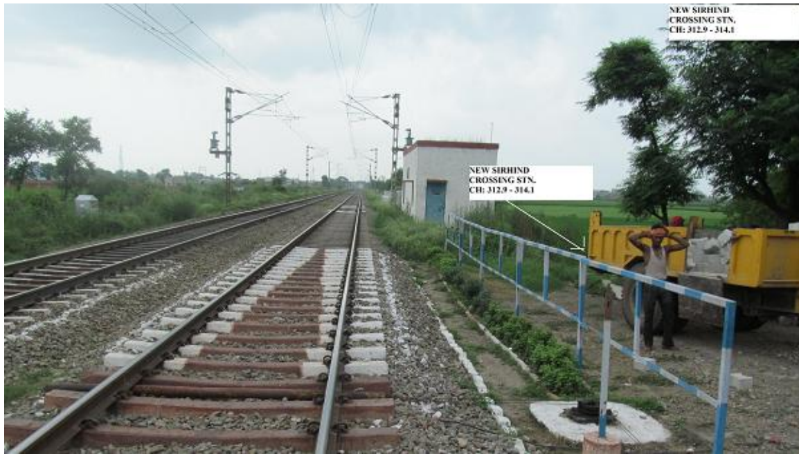
Figure 2.14 : Site for New Sirhind Crossing Station
