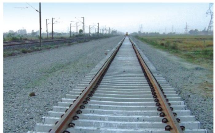
Track Linking at CH 56+700 on Eastern Corridor
