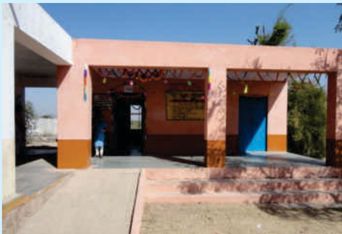
Computer Lab - Govt. Sec. School in Bedal, District-Pali in Western Corridor
