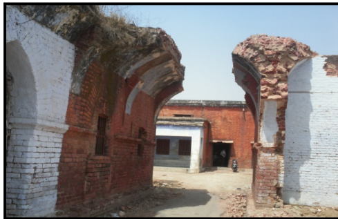
Photo :- 1 View of Archeological Monuments, Balai Kot or Upper Fort, Bulandshahr
