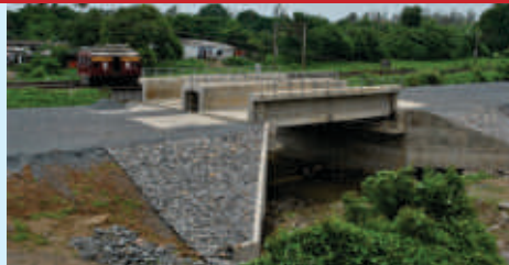
Bridge No. 230 at km in section 149/28-30 in Valsad District of Gujarat
