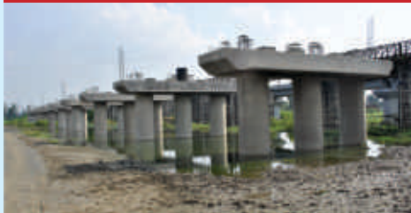
Bridge No. 400 at km in section 238/5-11 in Navsari District of Gujarat
