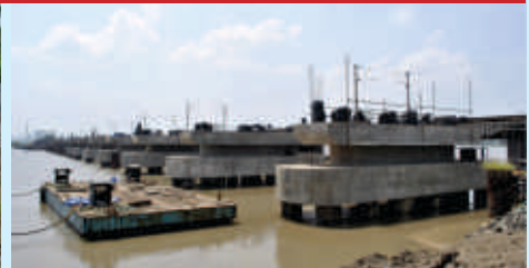
Bridge No. 93 at km in section 70/12-26 in Thane District of Maharashtra
