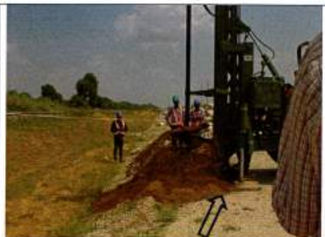
Wooden plank placed below the rest pad of outriggers
