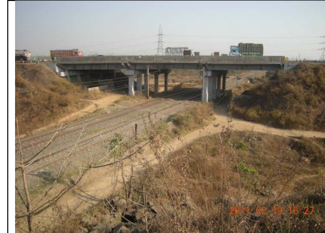
(3) ROB near Ulhas River (To be reconstructed)
