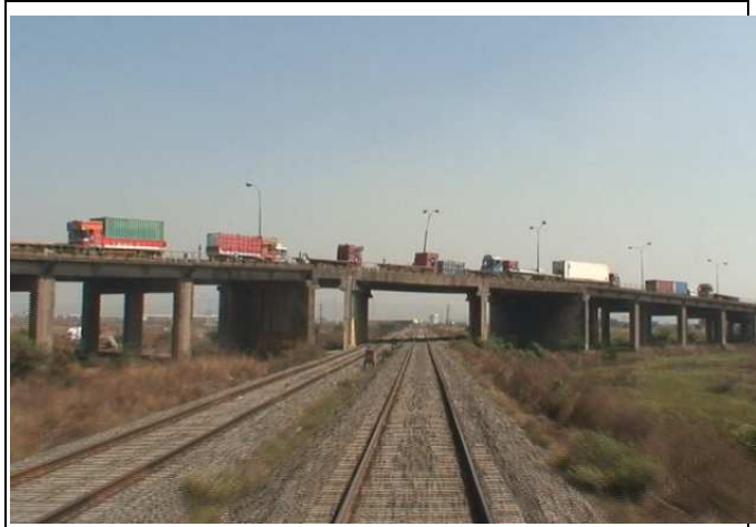
(1) ROB on JNPT Approach (To be reconstructed)
