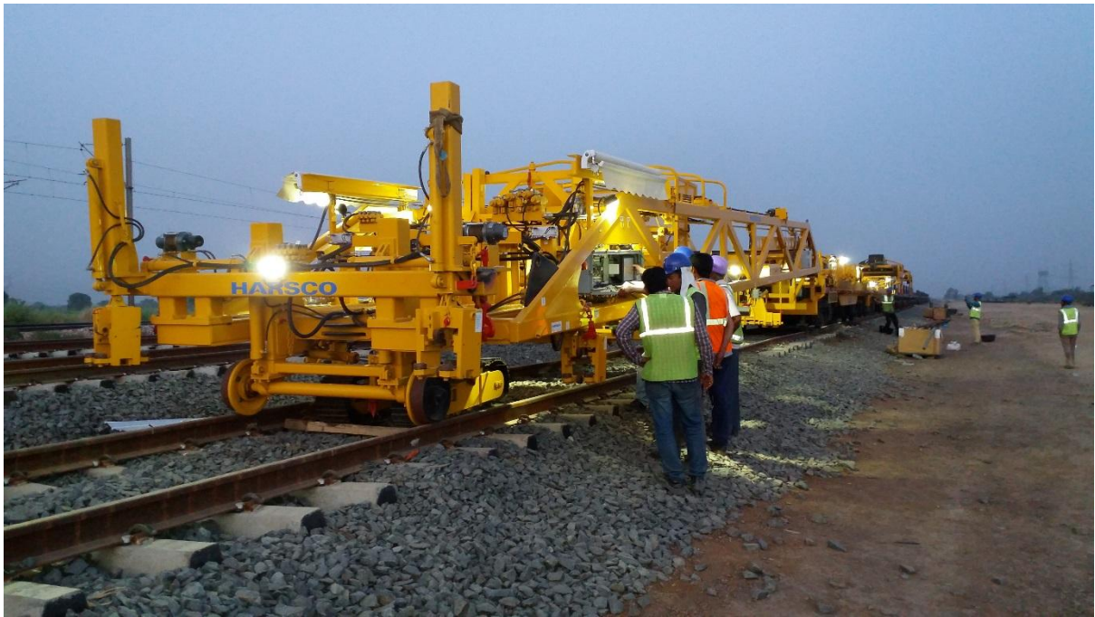
Work on DFC on full swing, New Track Laying (NTC) machine at Bhadan in Eastern DFC
