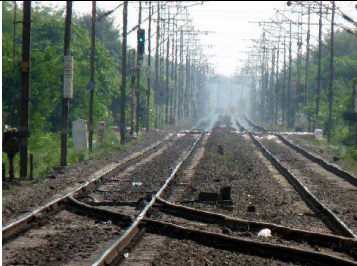
IR line atMakarpura Station
