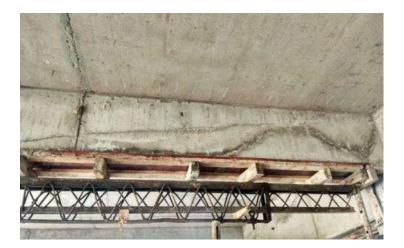
A cold joint or a poorly located and formed construction joint creates a plane of weakness in the concrete element and can adversely affect the durability of RCC/PSC elements. This defect is unlikely to be serious in itself unless accompanied by one of the serious defect listed above. However, if identified early, it can be rectified well in time
