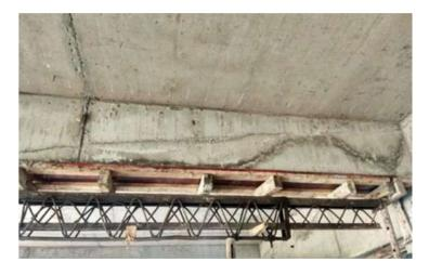
A cold joint or a poorly located and formed construction joint creates a plane of weakness in the concrete element and can adversely affect the durability of RCC/PSC elements. This defect is unlikely to be serious in itself unless accompanied by one of the serious defect listed above. However, if identified early, it can be rectified well in time to prevent it from becoming serious later on.
