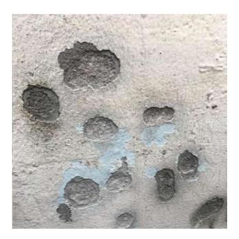
Blister and pop outs are very local defects and indicated by an irregular cavity on the concrete surface. It is typically caused by removal of coarse aggregate (or a foreign material or large air void) from concrete surface. This being a very local and superficial defect, surface repair is usually adequate. The location of blister should be recorded.
