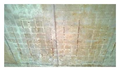
e. SURFACE ABRASION / DUSTING: In bridges, abrasion of concrete is generally noticed in the foundation and substructure which are subject to strong water currents. Dusting is a phenomenon associated with poor concrete in the top surface of a slab. Such a situation is unlikely to occur in a Railway Bridge. Abrasion will manifest by exposure of coarse aggregate or other marks on the surface of concrete (pier, well & pile cap and floor aprons). The location and extent of abrasion should be noted.
