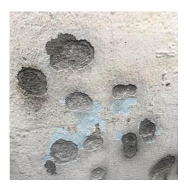
Blister and pop outs are very local defects and indicated by an irregular cavity on the concrete surface. It is typically caused by removal of coarse aggregate (or a foreign material or large air void)
