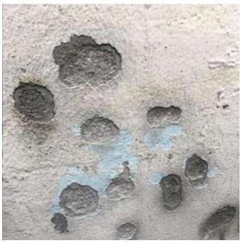
Blister and pop outs are very local defects and indicated by an irregular cavity on the concrete surface. It is typically caused by removal of coarse aggregate (or a foreign material or large air void) from concrete surface. This being a very local and superficial defect, surface repair is usually
