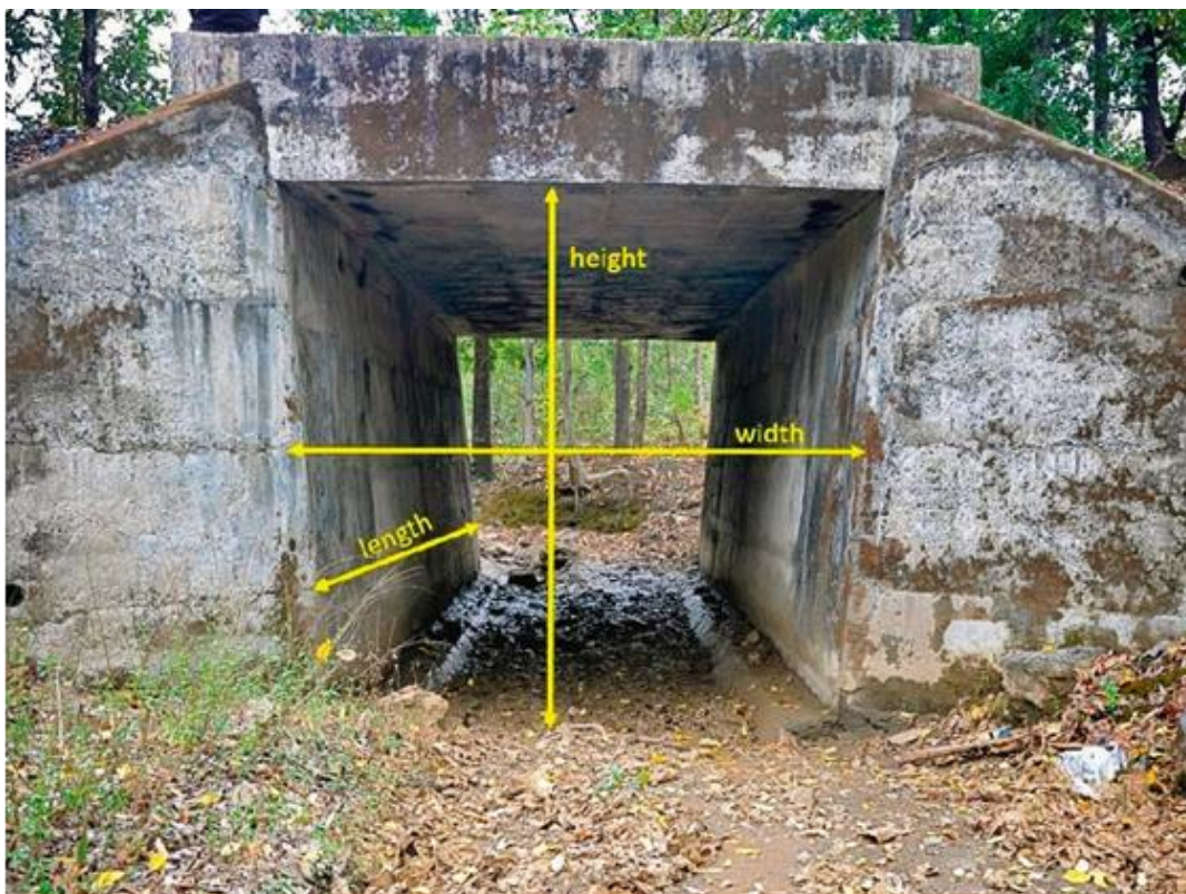
Figure No. 2.1 . Dimensions of an Animal underpass determining its openness.
