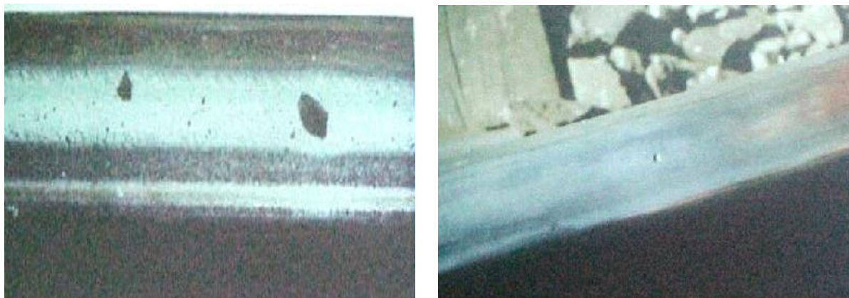
FIG. 48 : 301 - DAMAGE TO RAIL BY BRUSHING OR ARCING
